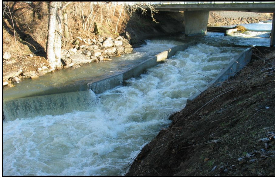
Figure 15: Photo of completed fish ladder at Gose Street during high flows.
