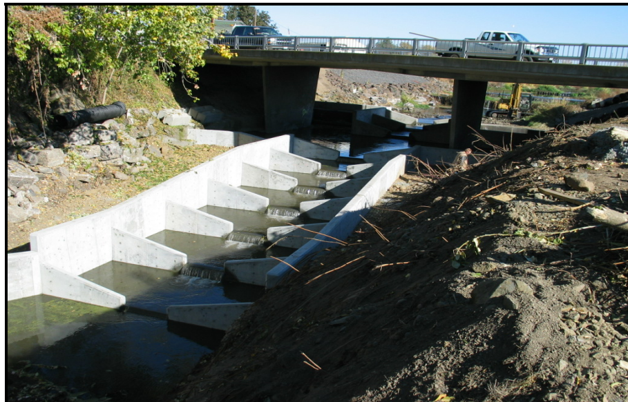
Figure 14: The photo was taken in late October of 2006 shortly after both new fish ladders were
