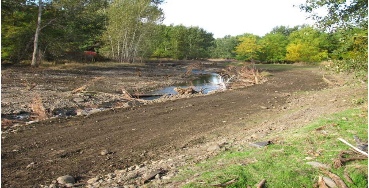
Figure 5: Looking downstream near the entrance of the newly constructed floodplain and side-channel. Large wood can be seen along the channel margin and within the floodplain along the left bank. Following construction, all disturbed areas of the project area were planted with several thousand native trees and shrubs.
