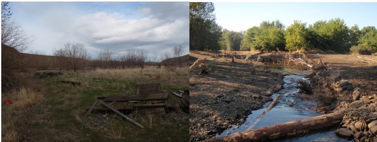
Figure 5: Looking downstream near the entrance of the newly constructed floodplain and side-channel. Large wood can be seen along the channel margin and within the floodplain along the left bank. Following construction, all disturbed areas of the project area were planted with several thousand native trees and shrubs.
