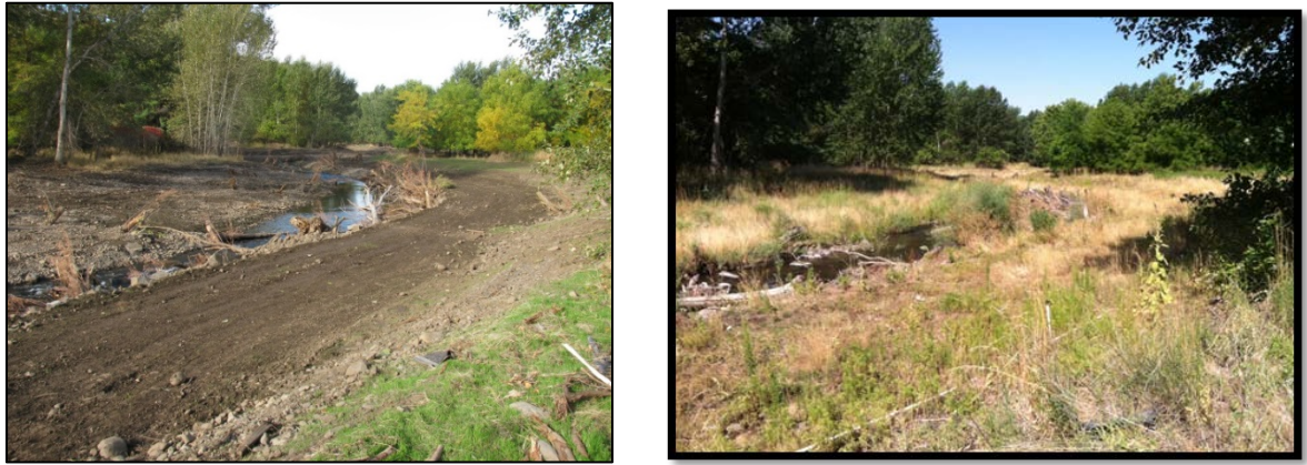
Figure 5: Looking downstream at the side channel following construction in 2011 left and same location two years later in June of 2013 on the right.
