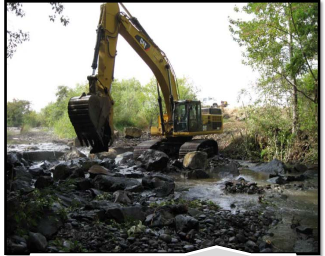
Photo looking upstream during the construction of the roughened channel
