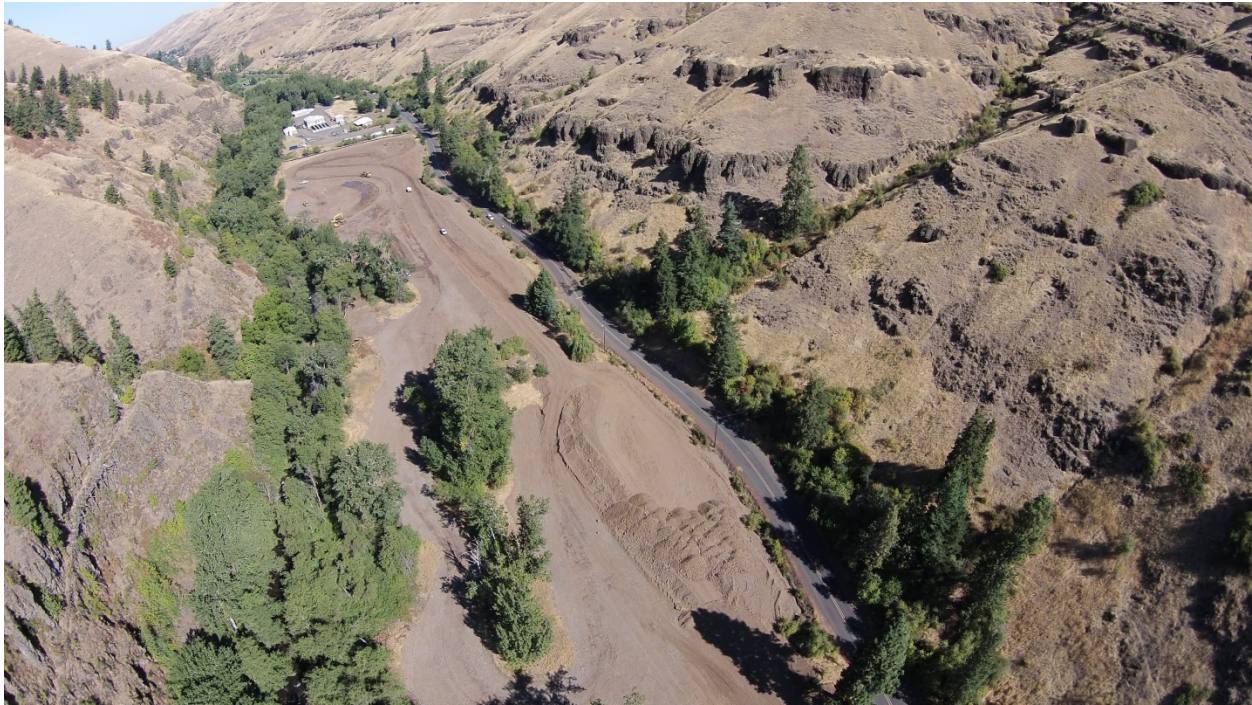
Figure 8: Aerial image of Kentch construction.
