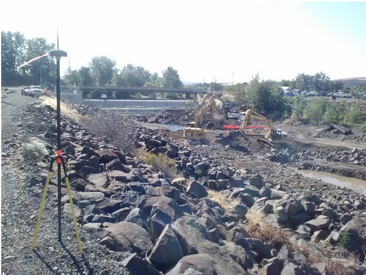
Figures 20-22: Nursery Bridge construction
