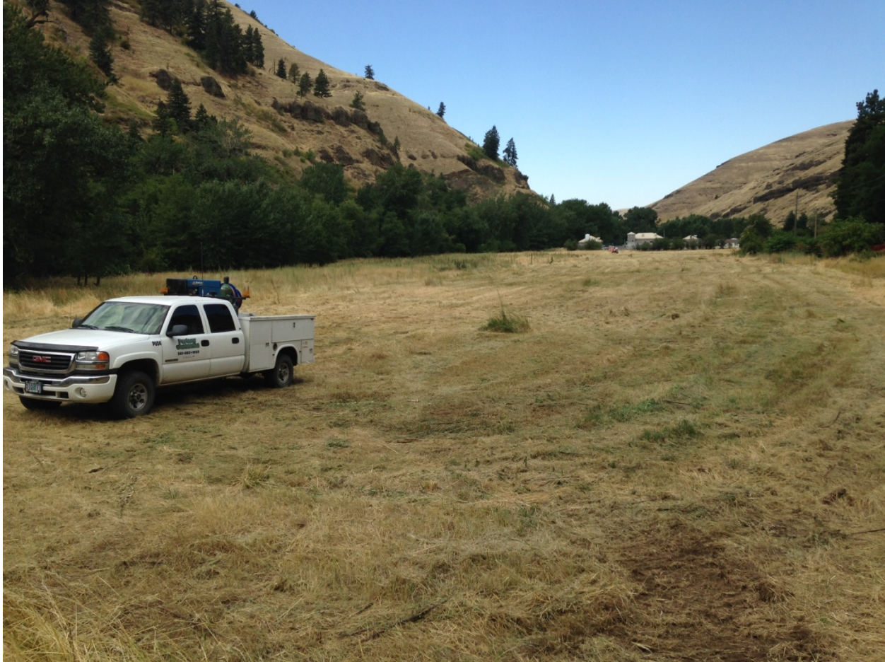
Figure 9: Kentch site on first day of construction, looking towards the hatchery.
