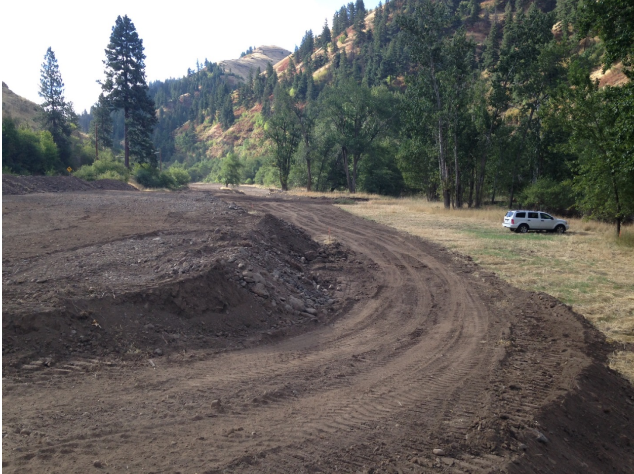
Figure 9: Kentch construction looking upstream
