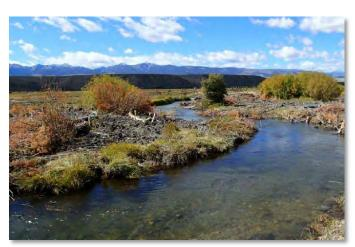
Bank fill stabilized with on-site harvested wetland sod immediately after construction; Big Springs Creek, ID
