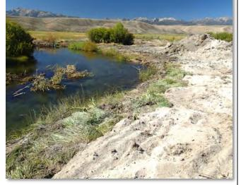
Strips of wetland sod harvested on-site used to retain unstable sandy bank fill immediately after construction; Big Springs Creek, ID
