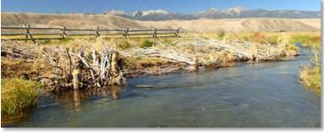
Willow clumps placed along the outside of a newly constructed meander bend to provide bank stability, instream structure, and cover immediately after construction; Big Springs Creek, ID.
