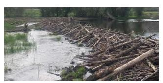
Figure 25. Treatment: Floodplain spanning structure designed to emulate a relic beaver dam
