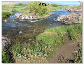
**Above:** Lemhi River, 1.5 years after construction of multi-threaded channel network using various bank and instream structure to split flow into many, short, narrow side channels.
