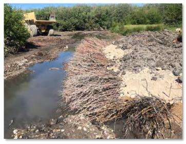
Willow brush layer during construction (Above) and immediately after construction (Below); Lemhi River, ID
