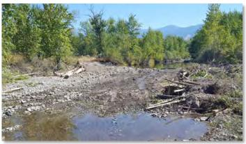
Constructed riffle during construction with wood structure installed on left bank (right side of photo); Lemhi River, ID
