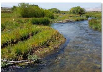
Strips of nursery-grown wetland sod placed over FESL bank treatment with potted willows between strips 1 year after construction; Big Springs Creek, ID
