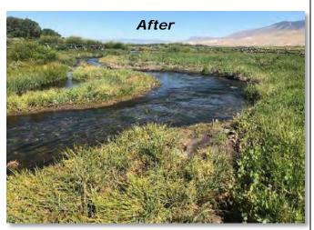
Big Springs Creek 1 year after construction; Width-to-depth ratio reduced by over 50% using FESL on both banks
