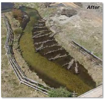
6 months after construction; fine sediment deposition observed between willow weaves; effective channel width reduced by approximately 50%
