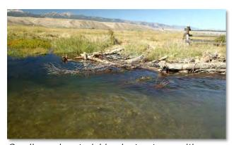
Small wood material bank structures with excavated scour pool immediately after construction; Big Springs Creek, ID
