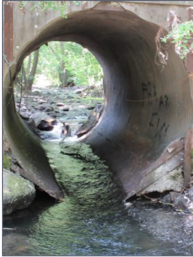
Figure 33. Culvert with no step, Unit 15, under a private road crossing.
