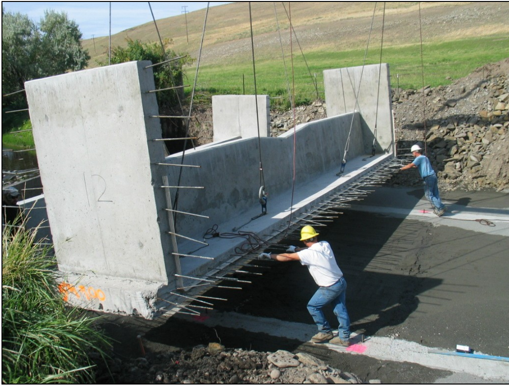
Figure 29. Moving Fishway Section Into Place
