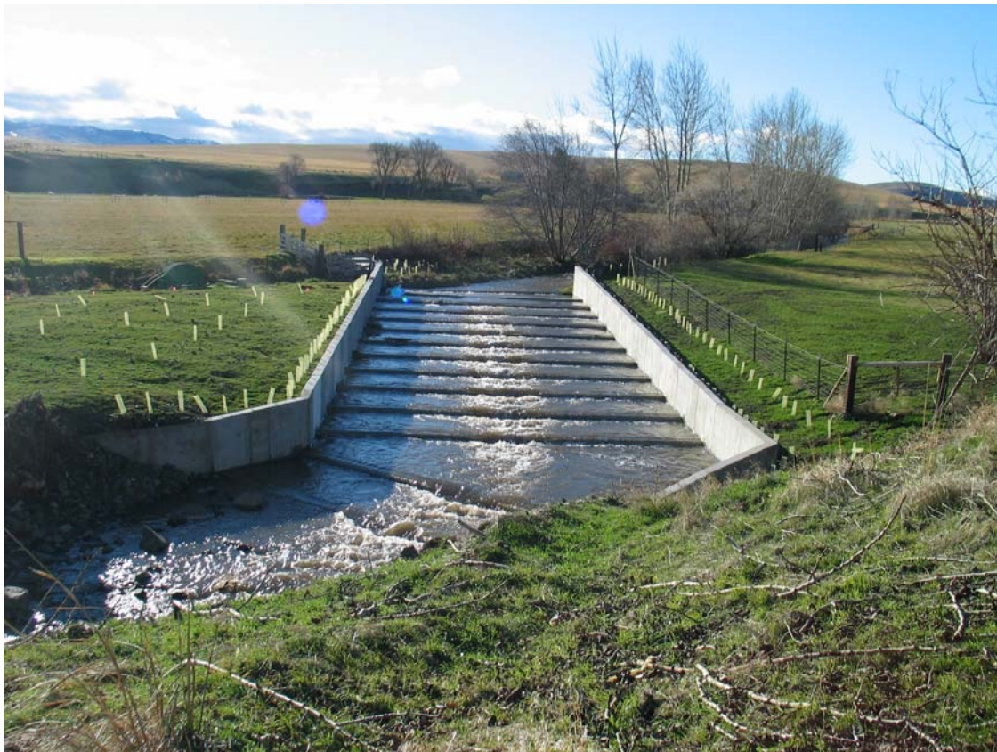
Figure 30. Hoeft Dam Post Construction
