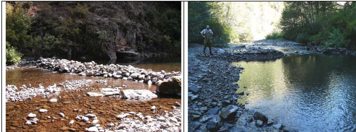
Figure 17. Recreational Dam on SF Umatilla River (left); SF Umatilla River Post Dam Removal (right)
