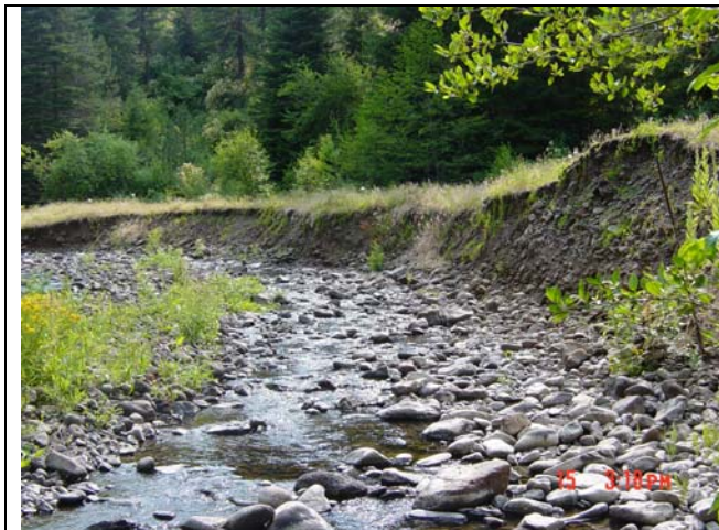
Actively Eroding Bank and High Terrace
