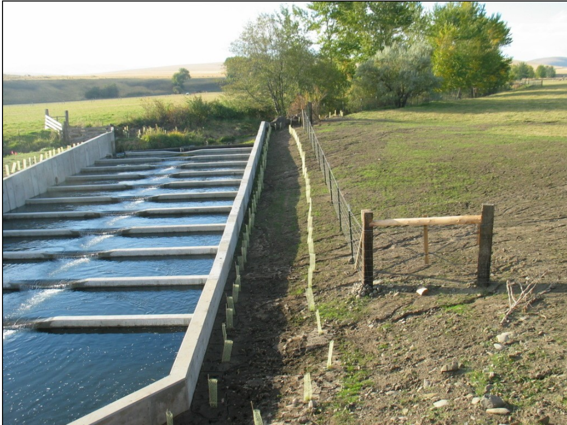
Figure 31. Hoeft Passage Rectification Project Showing Sloped Bank and Plantings
