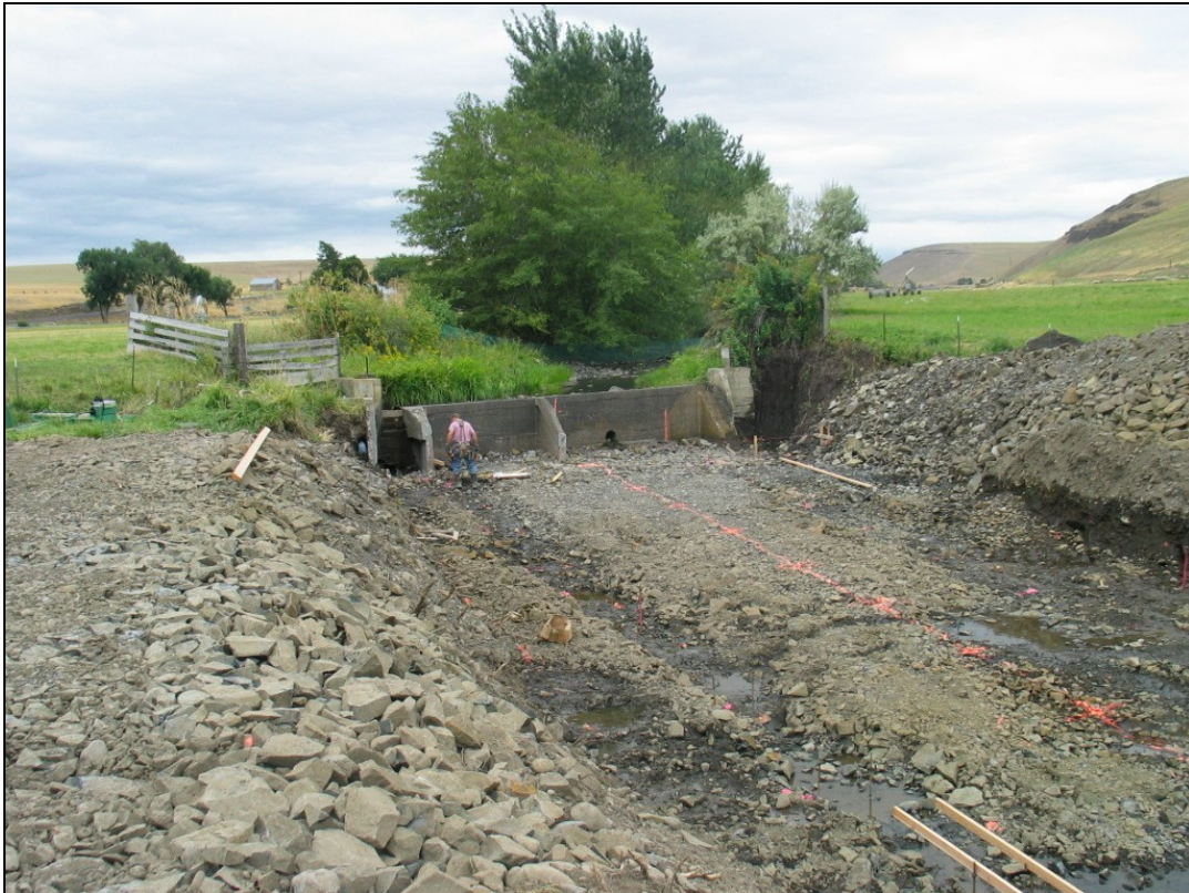
Figure 27. Hoeft Dam – Preparation of Substrate for Fishway Base
