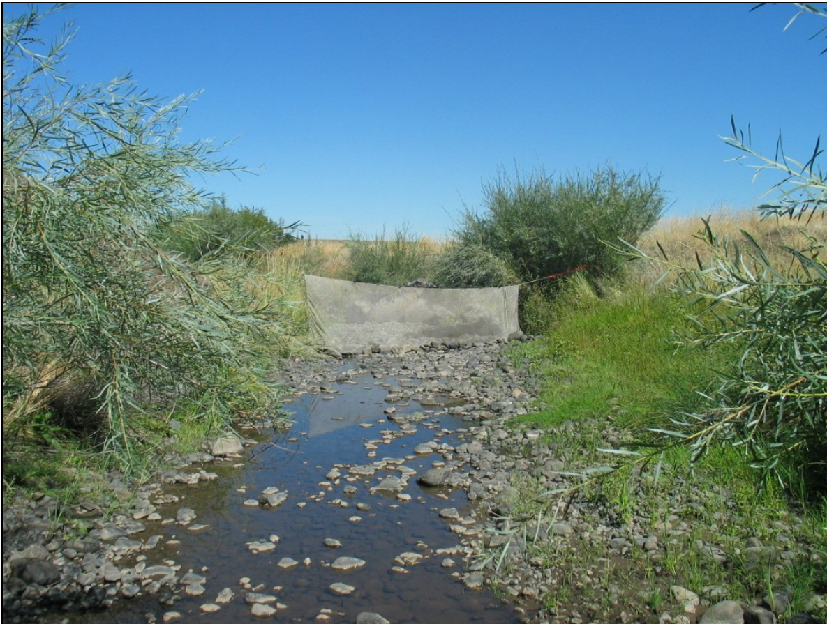
Figure 26. Blocknets Used to Keep Fish From Reentering Construction Site
