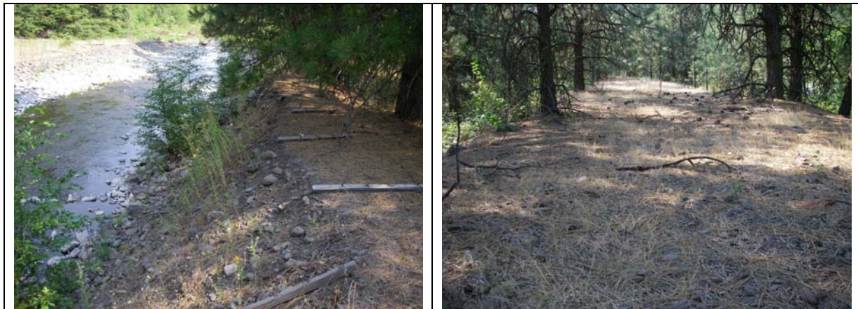
Figure 20. Example of Levee Along Meacham Creek
