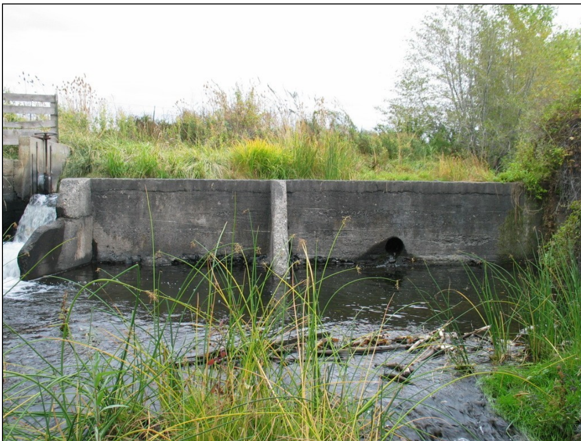
Figure 24. Hoeft Dam on West Birch Creek, RM 2.7 Prior to Rectification
