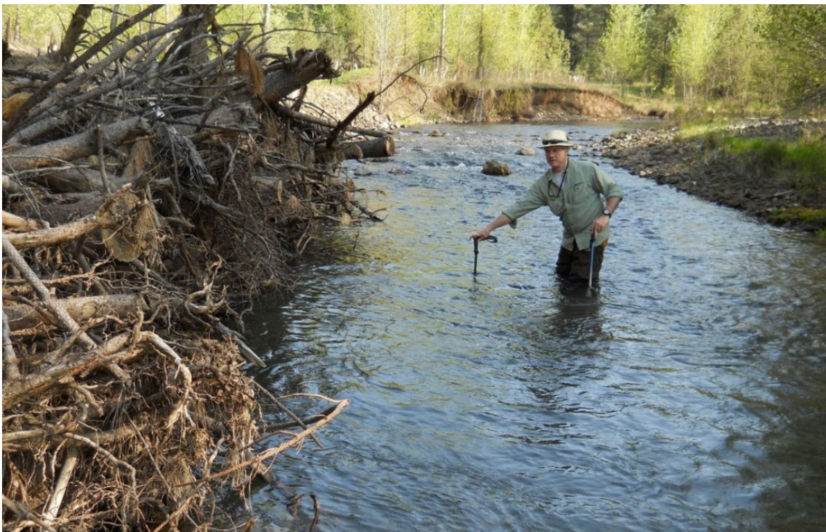
Figure 26. Example scour pool formation in front of a crib jam.
