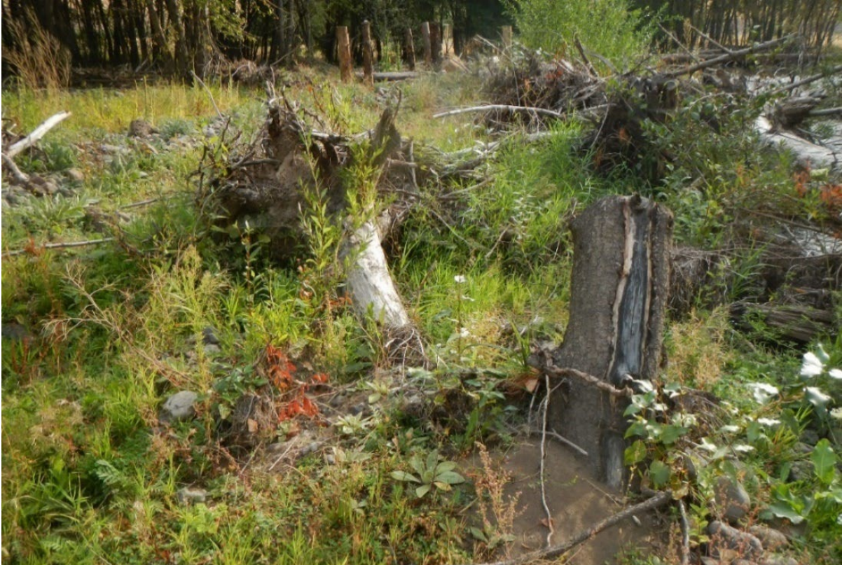
Figure 25. Example of a debris catching log array placed on a gravel bar to trap wood and promote sediment deposition and vegetative colonization.
