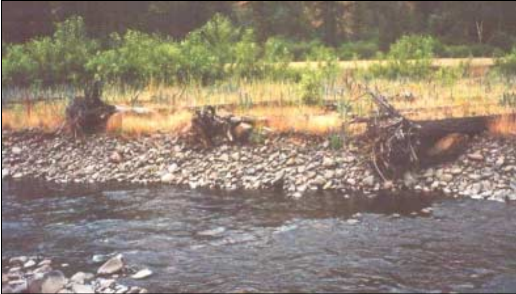
Figure 28. Log/boulder structures near river mile 3.6 rafted onto a low terrace during a high flow.
