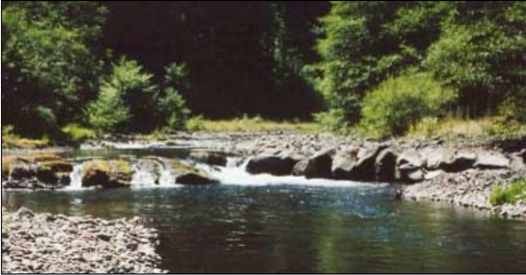
Figure 33. Cabled boulders added to the top of a bedrock cascade now prevent upstream passage of juvenile fish during summer low flow. Site number #7 in Appendix D.
