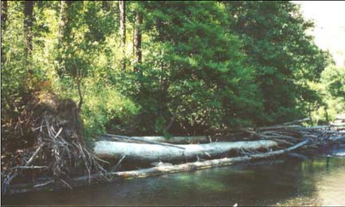
Figure 29. Well-designed log/boulder structure (# 26 at river mile 2.25) that creates year-round cover and pools.
