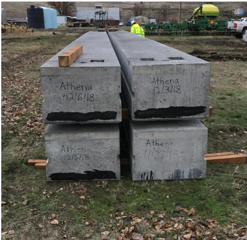
Figure 14. Precast, prestressed concrete bridge deck planks delivered to Mission, OR, in December 2018.
