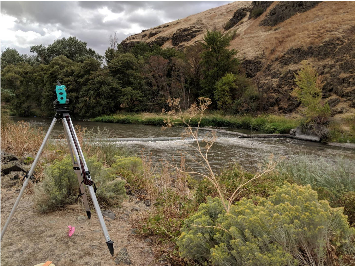
Figure 17. CTUIR staff conducting total station surveys of the Taylor Diversion Dam to support BPA engineering staff in designing the removal of the dam.
