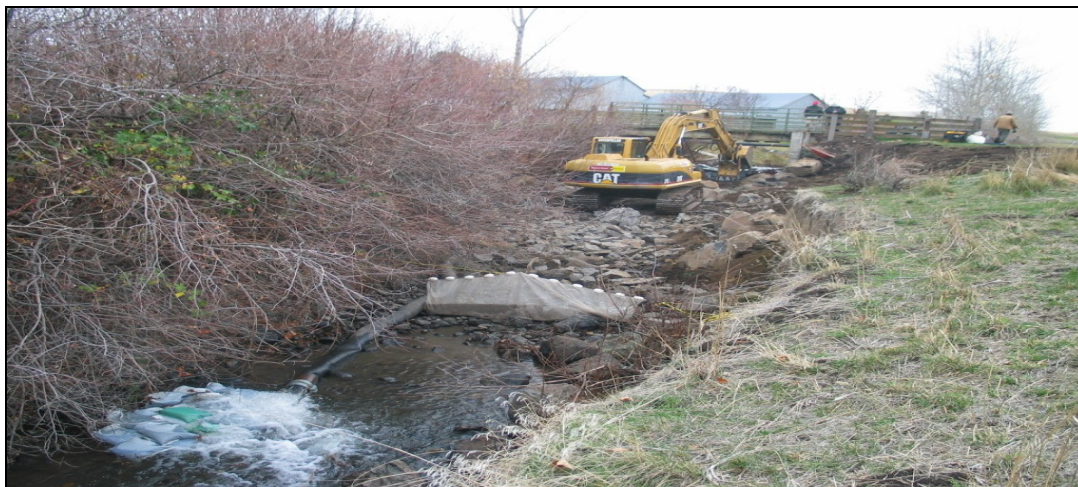
Figure 30. Dewatering and Site Isolation Method, West Birch Creek, RM 3.2, Cunningham Bridge
