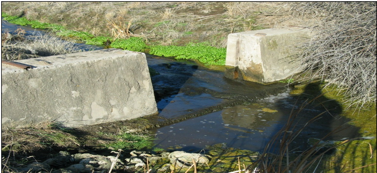
Figure 26. Greasewood Creek Fish Passage Barrier, RM 0.4 Post Rectification
