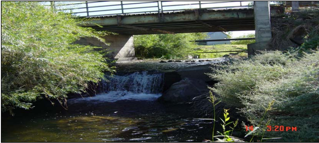
Figure 28. Cunningham Bridge on West Birch Creek, RM 3.2 Prior to Rectification
