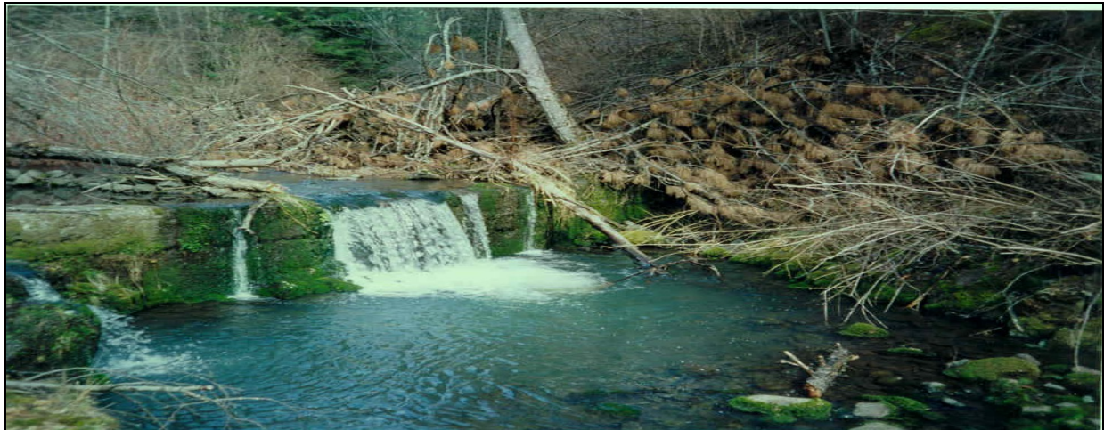
Figure 23. Camp Creek Fish Passage Barrier, RM 0.3 Prior to Rectification
