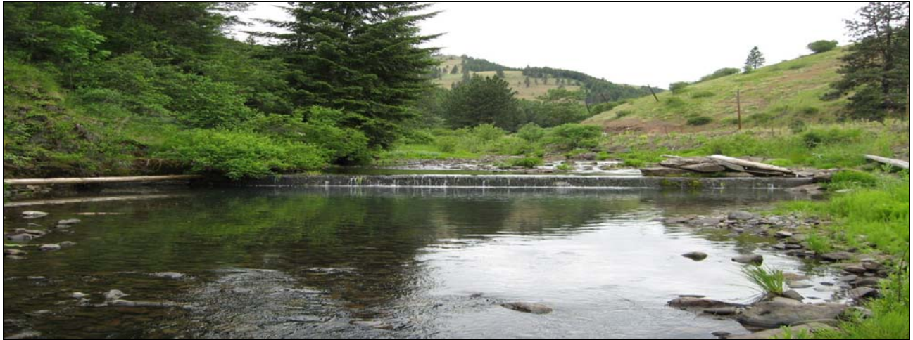
Figure 20. Meacham Creek Fish Passage Barrier, RM 20.2 Prior to Rectification
