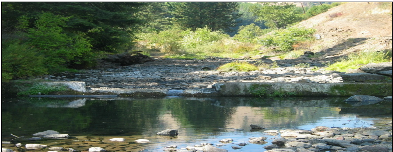
Figure 21. Meacham Creek Fish Passage Barrier, RM 20.2 Post Rectification
