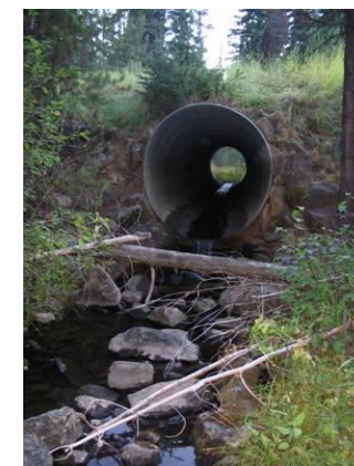
Passage barrier on Sponge Creek
