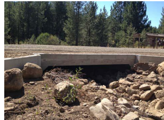
Ten Cent Creek Culvert Replacement #3
