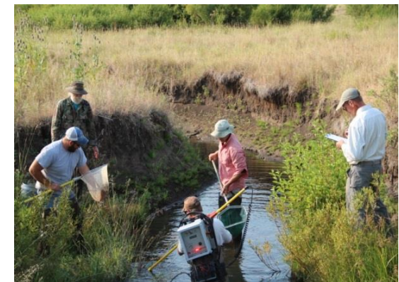
Fish Salvage prior to the Fox Creek USACE Channel Realignment
