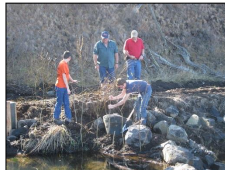
Placing the footer log of a large wood structure to improve streambank stability in Granite Creek (right)
