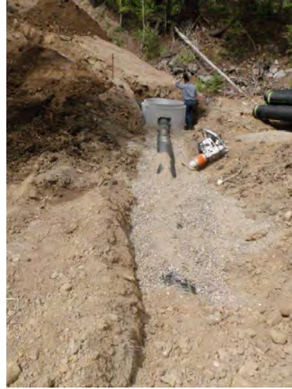
Figure 24. Photographs showing the intake adjacent to the mine audit (left) and pipe and manhole being bedded (right).
