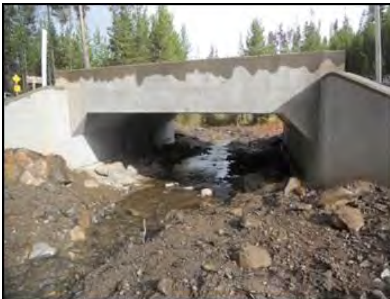
Figure 21. Pre-cast concrete bridge which replaced a round 4' in 2013.
