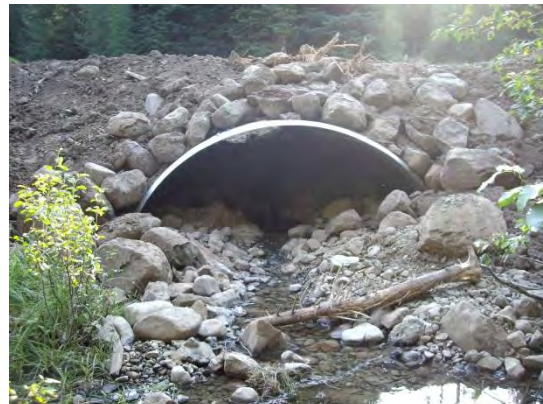
Figure 11. Original upper Ten Cent Creek culvert (left) replaced by a bottomless arch on footers in 2012.
