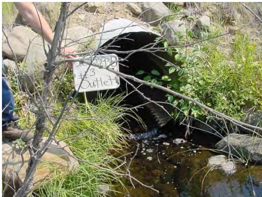
Figure 11. Original upper Ten Cent Creek culvert (left) replaced by a bottomless arch on footers in 2012.
