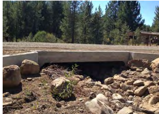
Figure 9. Original lower Ten Cent Creek culvert (left) replaced by a pre-cast concrete bridge in 2012.
