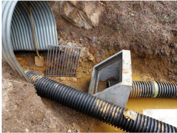
Figure 24. Photographs showing the intake adjacent to the mine audit (left) and pipe and manhole being bedded (right).
