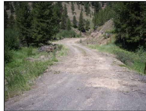
Culvert across Bull Run Creek
