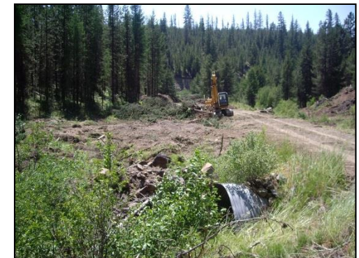
Culvert across Deep Creek
