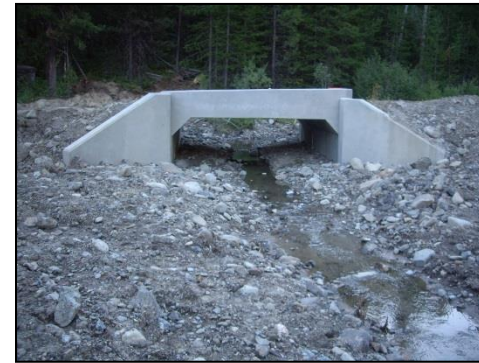
Left - Completed pre-cast concrete bridge across Bull Run Creek.
