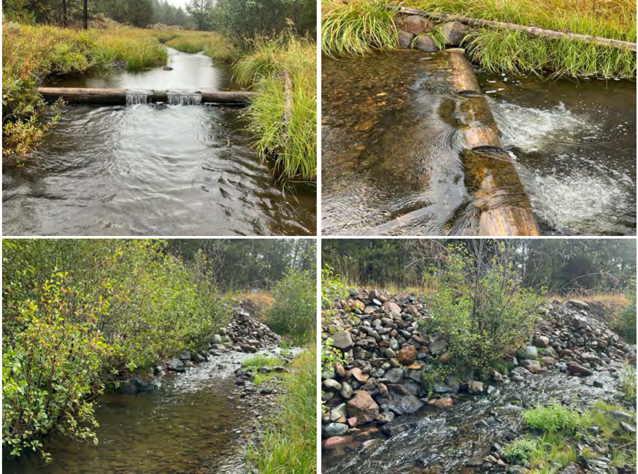
Figure 9. Images of placed wood and an armored bank located on Bull Run Creek.
