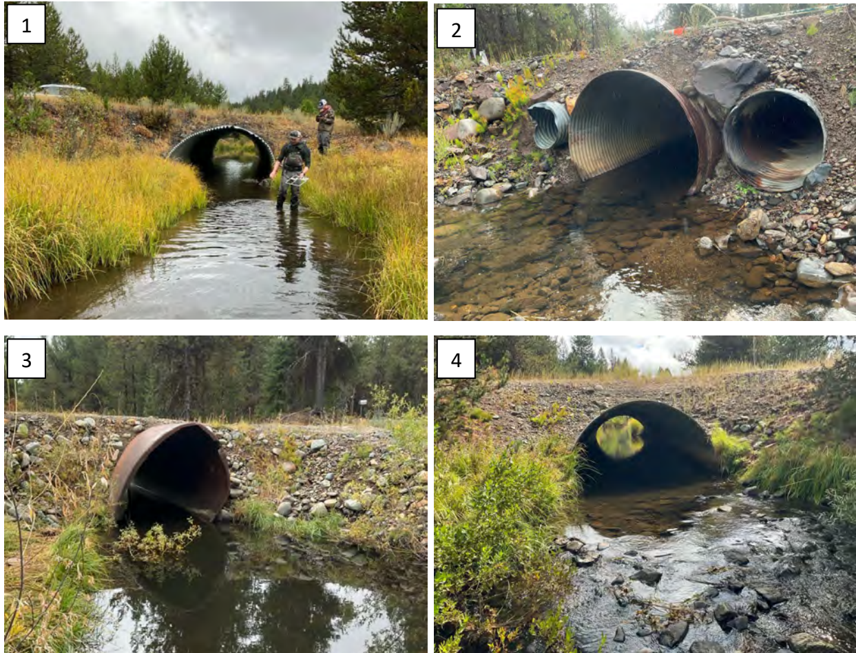
Figure 8. Images of culverts located along Bull Run Creek project area (1 through 4).
