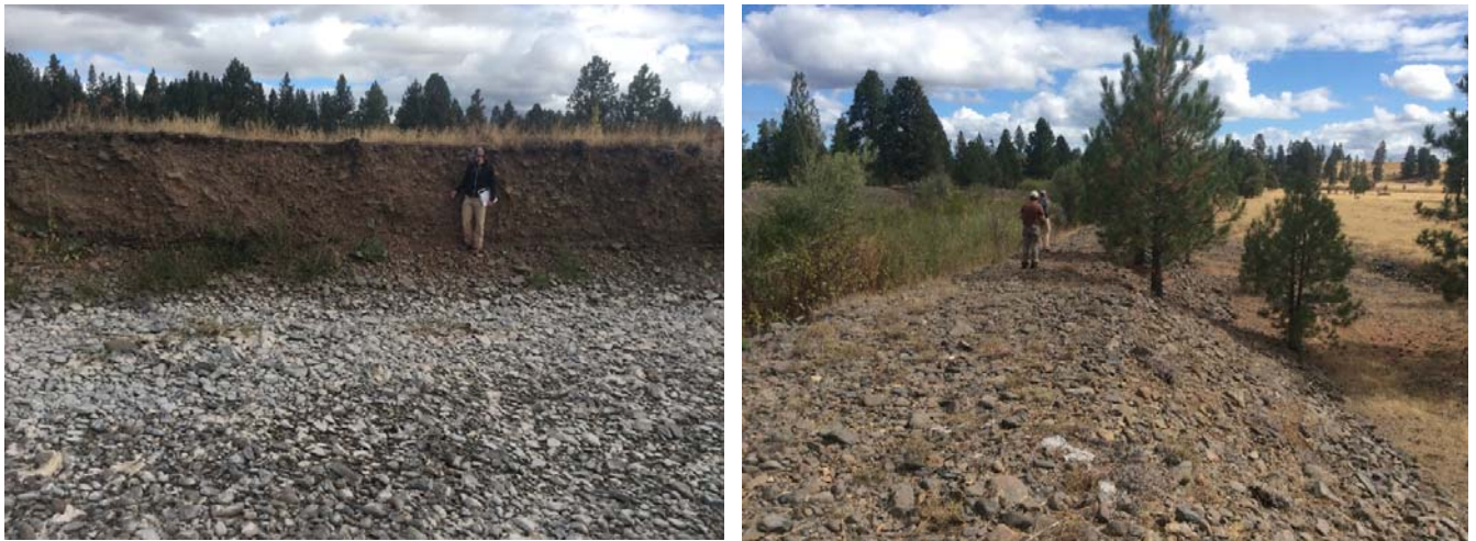
Figure 13. Eroding levee along Camas Creek at RM 14.2 (left) and intact left bank levee at RM 14.4 (right).
