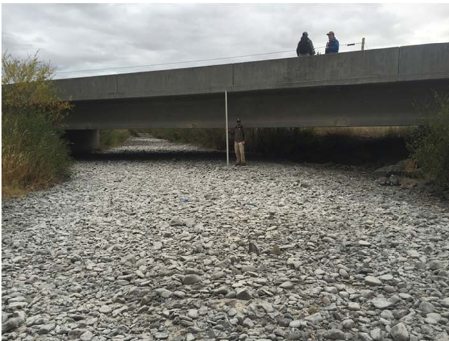
Figure 12. Camas Creek aggradation at the Camas Street Bridge (Sep. 2015).
