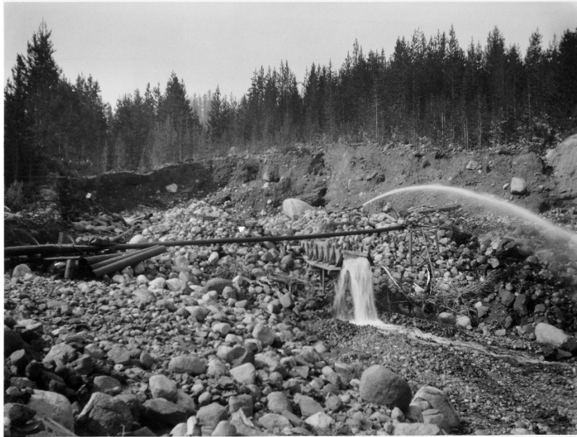
Figure 12. Hydraulic sluicing in the UNF. Photo from John Guthrie, circa 1930.
