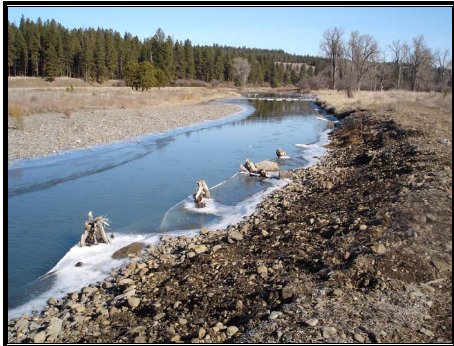
Longley Meadows, Grande Ronde Photo Point GR-3 10/04. Post-phase 2 construction. (Note rootwad revetments, streambank contouring, and large pool habitat development)
