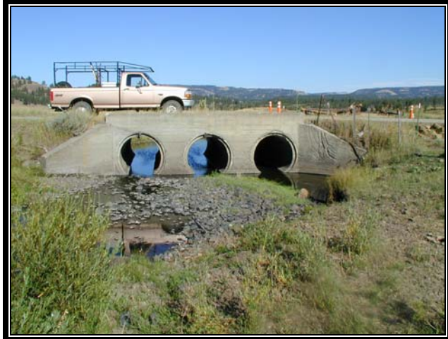
Pre-project triple culvert on McIntyre Road. Existing structure was severely undersized for McCoy Creek.
