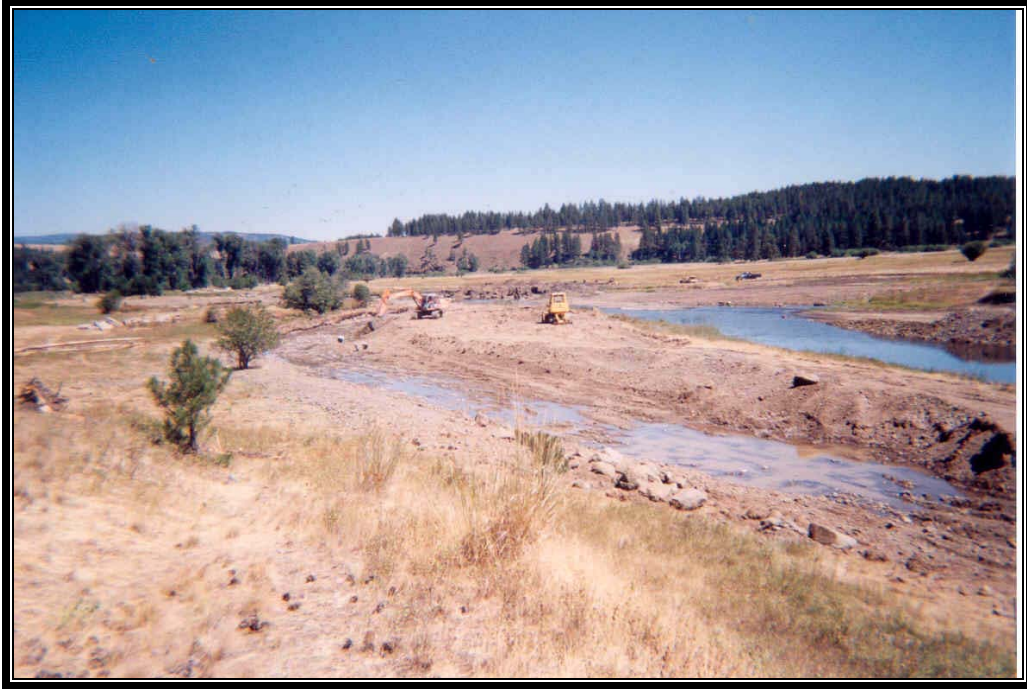
Mainstem Grande Ronde Project – photo illustrates the construction of new meander channel just upstream of Bear Creek. The excavator is shaping the bankfull channel form and right bank. In this photo the Grande Ronde River is still flowing in its old location along the right side.
