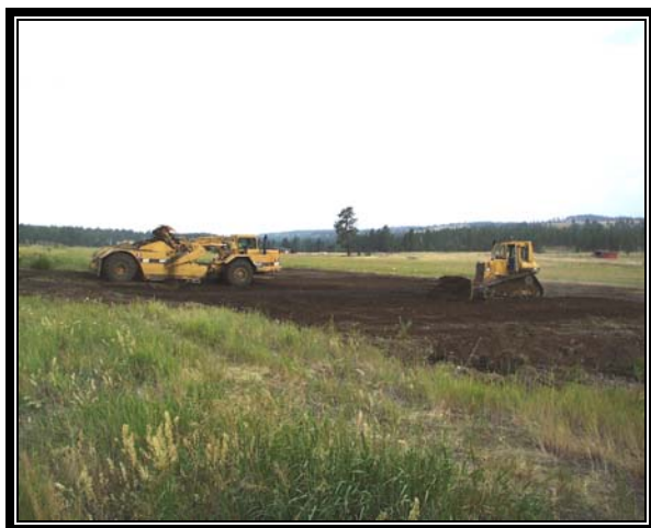
Phase 2 McCoy Creek channel construction. Photo illustrates use of large construction equipment including scraper loaders and track-mounted dozers.
