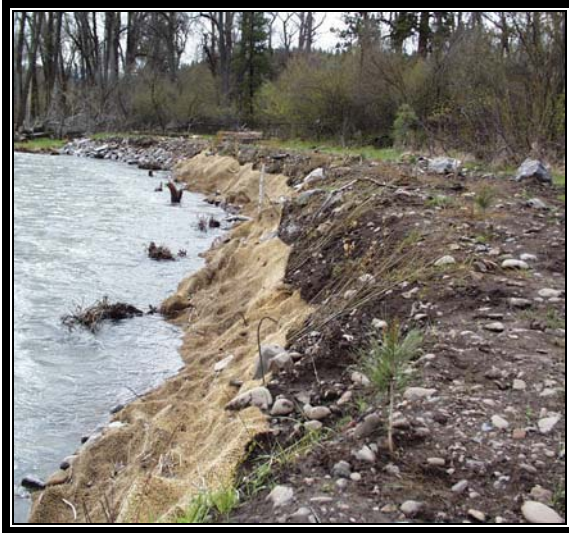
Mainstem GR Phase I Photo Point (Oct 99'). Streambank stabilization using rootwad revetments and bioengineering to meet landowner streambank stabilization objectives.
