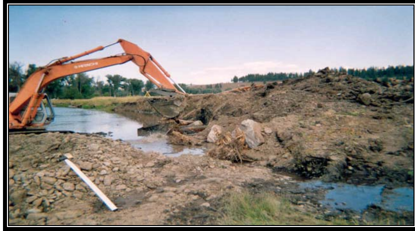
Mainstem Grande Ronde Project – photo shows the construction of a rootwad revetment along the right bank at site 4, just downstream of Bear Creek. Rootwads with 20-foot boles are placed on top of footer logs and then backfilled. The upper portion of the bank will be tapered back to a 4:1 slope.
