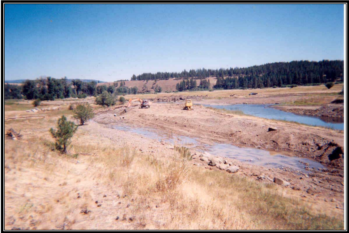
Longley Meadows, Mainstem Grande Ronde Project, Photo Point GR-5 – photos illustrate the construction of new meander channel just upstream of Bear Creek.
