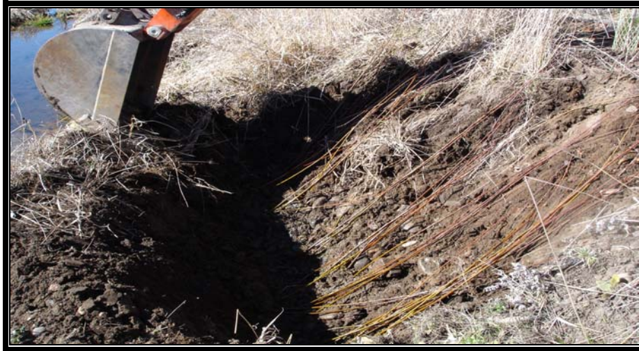
Mainstem Grande Ronde River – Shrub planting included mechanical installation of bundled, conditioned live willow whips. Strategy includes deep installation of material near water sources to facilitate recovery.
