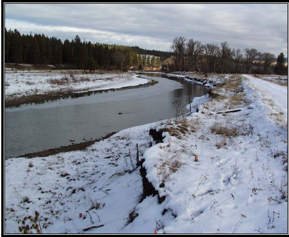
Longley Meadows, Grande Ronde Photo Point GR-3 10/04. Post-phase 2 construction. (Note rootwad revetments, streambank contouring, and large pool habitat development)
