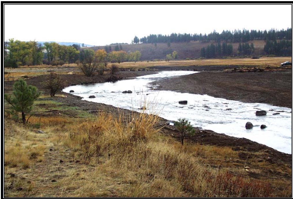
Mainstem Grande Ronde Project – photo illustrates post construction of new meander channel just upstream of Bear Creek. Channel diversion is complete and revegetation activities have been initiated.
