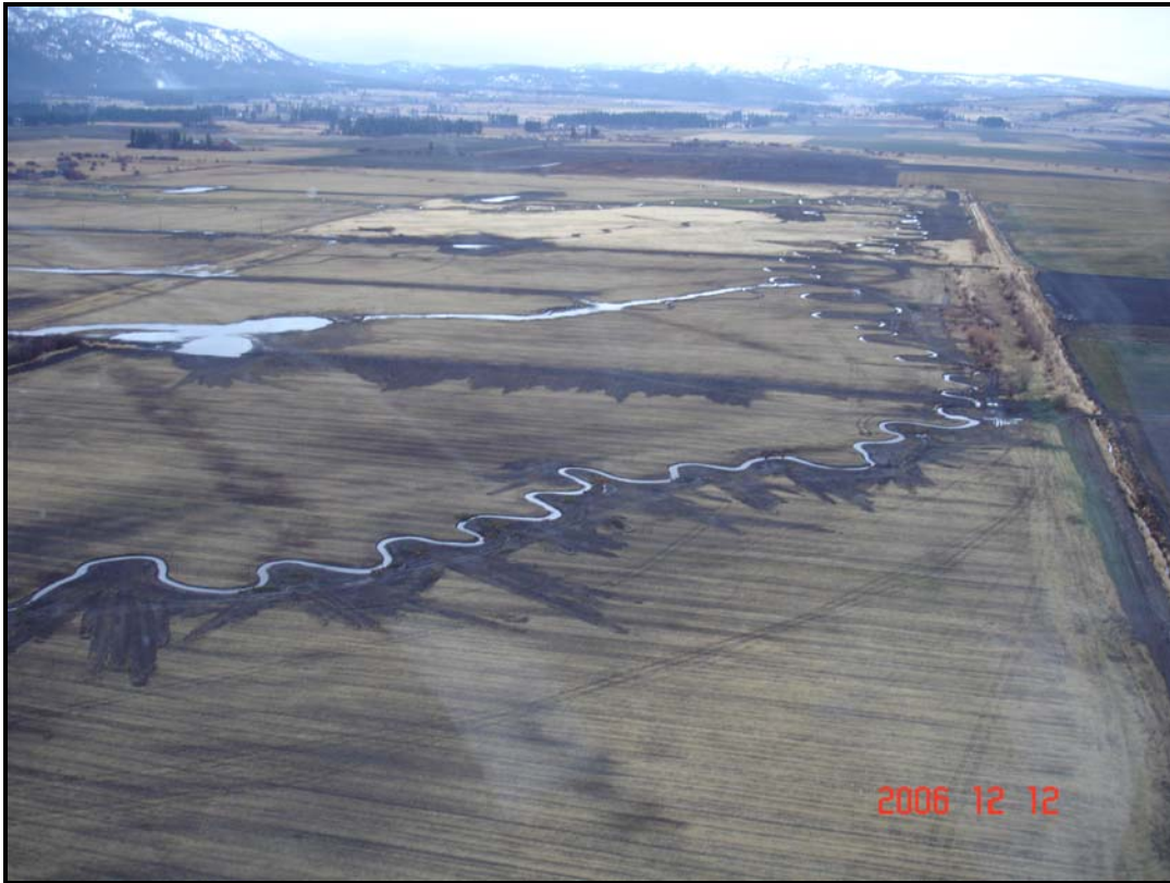
Upper reach of South Fork Willow Creek restoration channel viewing downstream towards confluence with End Creek restoration channel. Note large woody debris placement in channel and floodplain. December 2006
