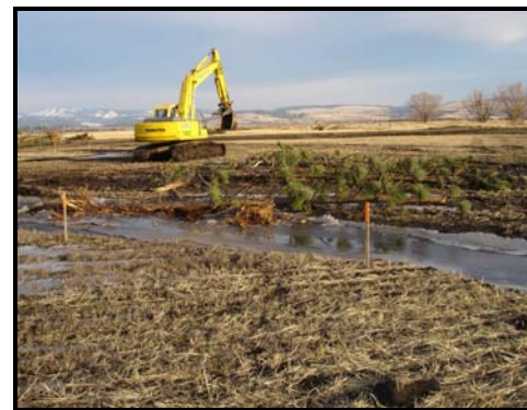
November 2006 photo illustrating wood placement along South Fork Willow restoration channel.
