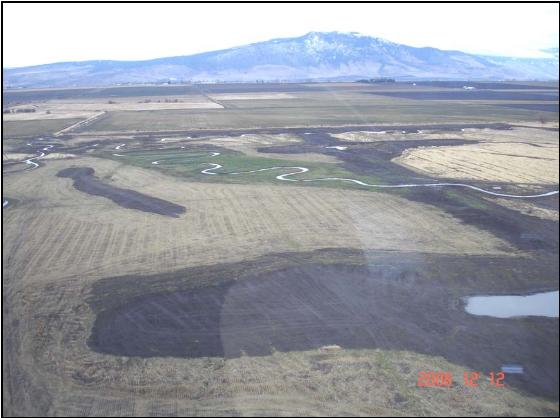
Lower End Creek Restoration Channel with floodplain pond in middle foreground. December 2006
