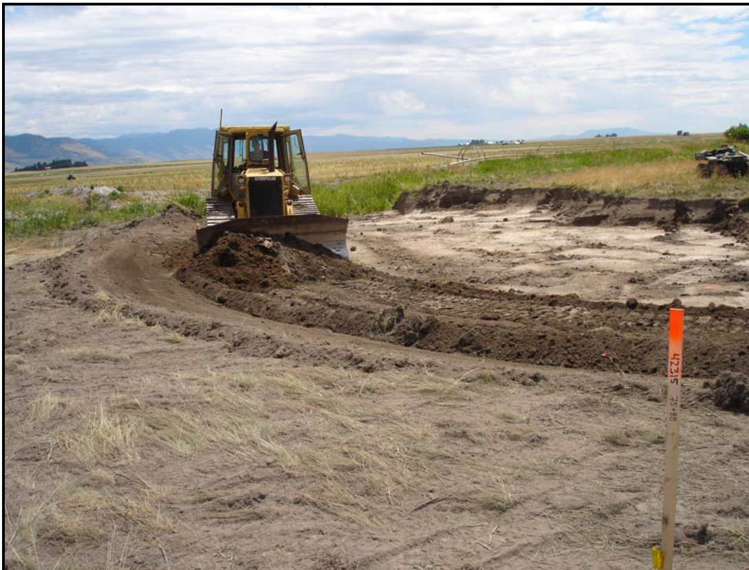
Initiation of channel construction on lower End Creek. December 2006
