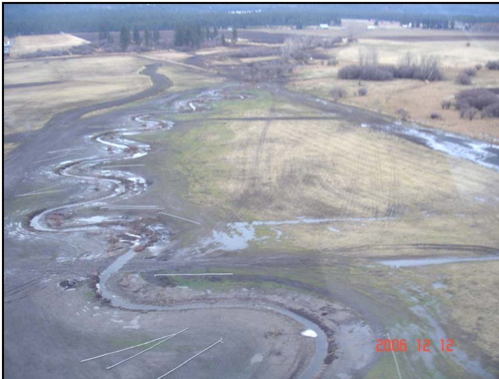
Upstream view of upper End Creek restoration channel. December 2006
