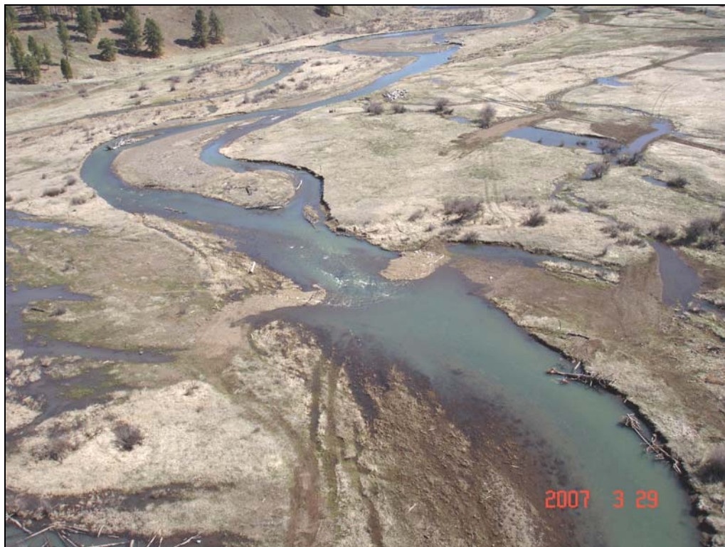
March 2007, Meadow Creek Restoration Project – Photo illustrates graded riffle weirs and large wood placement along Meadow Creek.
