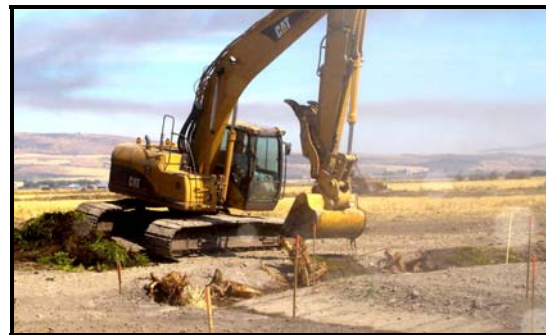
September 2006 photo illustrating rootwad revetment and installation of sedge/rush mats.
