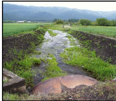
June 2003 Photos illustrate lower channelized End Creek. Extensive channelization in project area created unstable stream channels, excessive erosion, elevated water temperatures, loss of riparian and wetland vegetation, and poor fish habitat.
