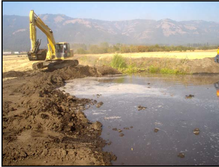
Floodplain pond construction. August 2006.
