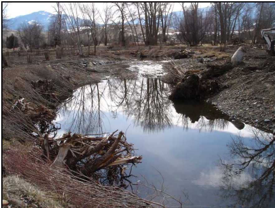
Upper project reach illustrating spring planting activities. Note whole tree and shrub planting in upper left of photo along floodplain. Willow whips in bottom foreground are temporarily stored in water prior to planting.
