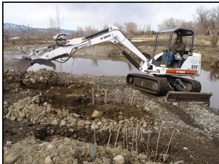
Gravel bar coyote willow trenching using a small track-mounted excavator
