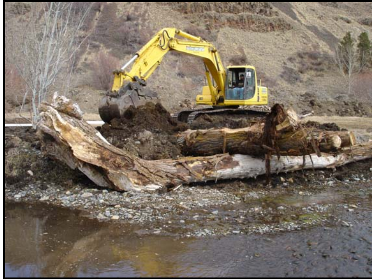
Large woody debris placement in conjunction with revegetation efforts. Project staff determined that completing wood placement prior to revegetation activities would minimize disturbance of planted and seeded materials
