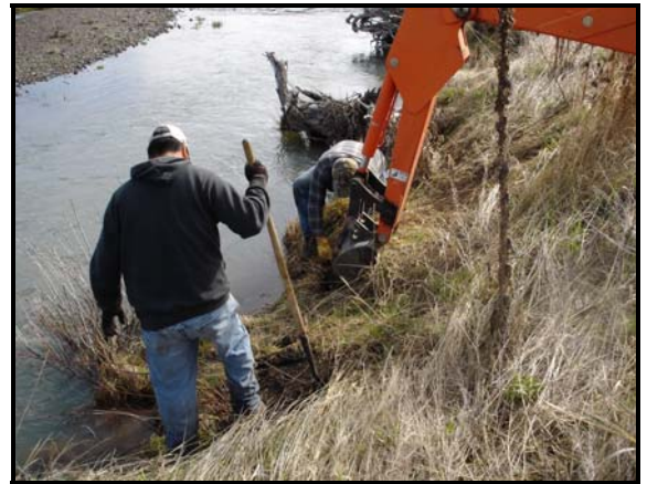
Mechanical installation of live willow whips. Track-hoe is utilized to excavate small trench to install pre-conditioned whips. Deep planting improves survival and facilitates establishment.
