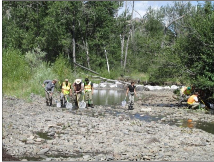
FIGURE 24 CREWS SALVAGING ROUGHENED CHANNEL. NOTE LARGE SUBSTRATE AND SHALLOW DEPTH.
