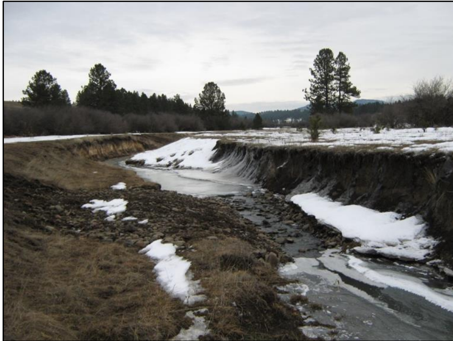
FIGURE 21 ONE OF THE PLUGS ALONG THE CHANNELIZED REACH OF GRAVES CREEK MADE FROM LEVEE MATERIAL REMOVED FROM THE ROCK CREEK FLOODPLAIN. TOP PHOTO WAS TAKEN LOOKING UPSTREAM IN 2013 AND BOTTOM PHOTO WAS TAKEN IN DECEMBER 2014 – 3 MONTHS AFTER CONSTRUCTION OF THE PLUG.
