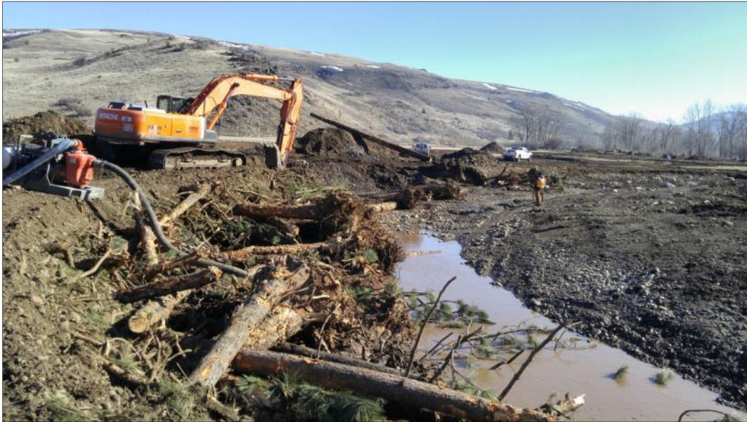
FIGURE 11 CONSTRUCTION OF DOWNSTREAM BEND STRUCTURE AT STATION 46+50.
