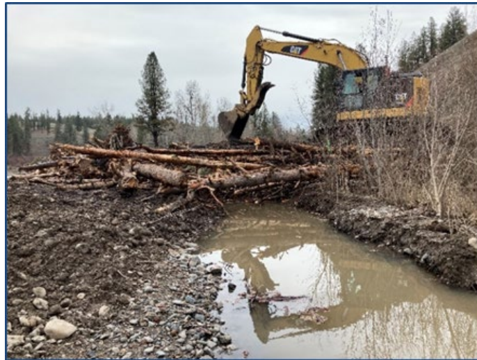
FIGURE 6 LARGE WOOD STRUCTURE IN SIDE CHANNEL 5
