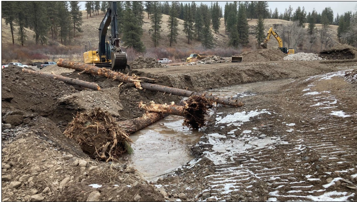
FIGURE 9 LARGE WOOD STRUCTURE CONSTRUCTION
