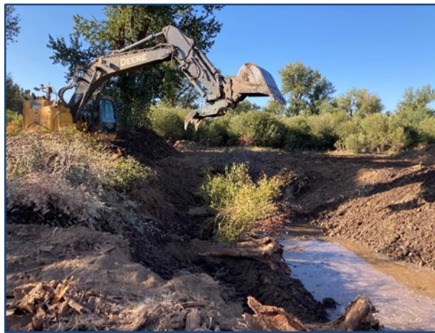
FIGURE 20 REPLANTING SALVAGED WILLOW CLUMPS, LONGLEY MEADOWS PROJECT
