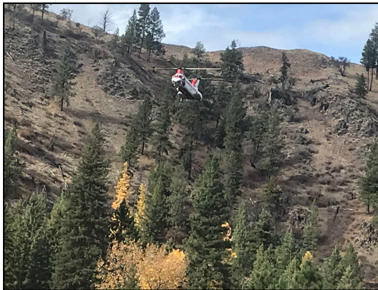
FIGURE 15 HELICOPTER BOULDER ADDITION
