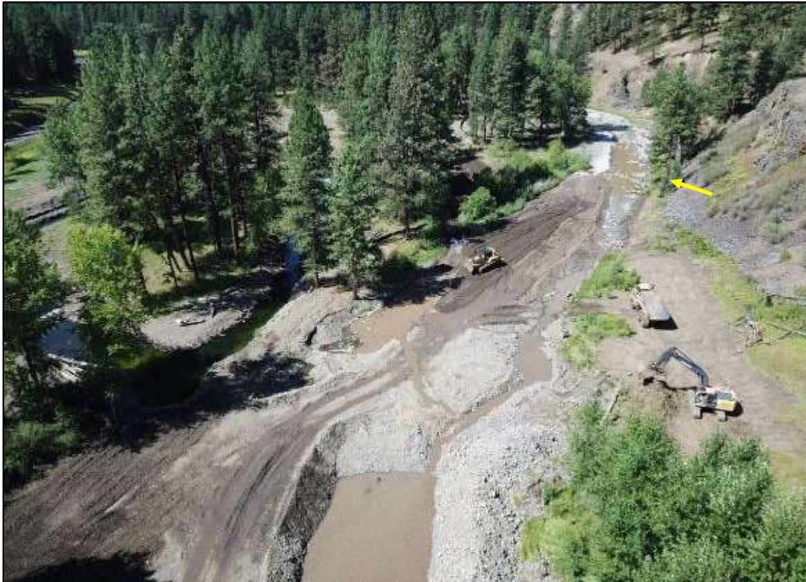
VIEWING DOWNSTREAM. STATIONING MC 37+00 – 42+00, SC2 AND MC CONFLUENCE
