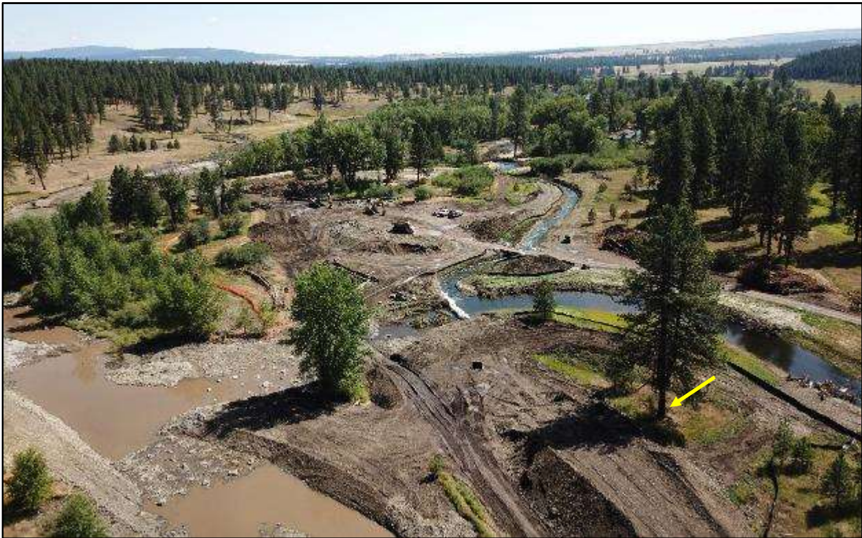
GROUND PHOTO POINTS – BEFORE (LEFT) AND AFTER CONSTRUCTION (RIGHT)
