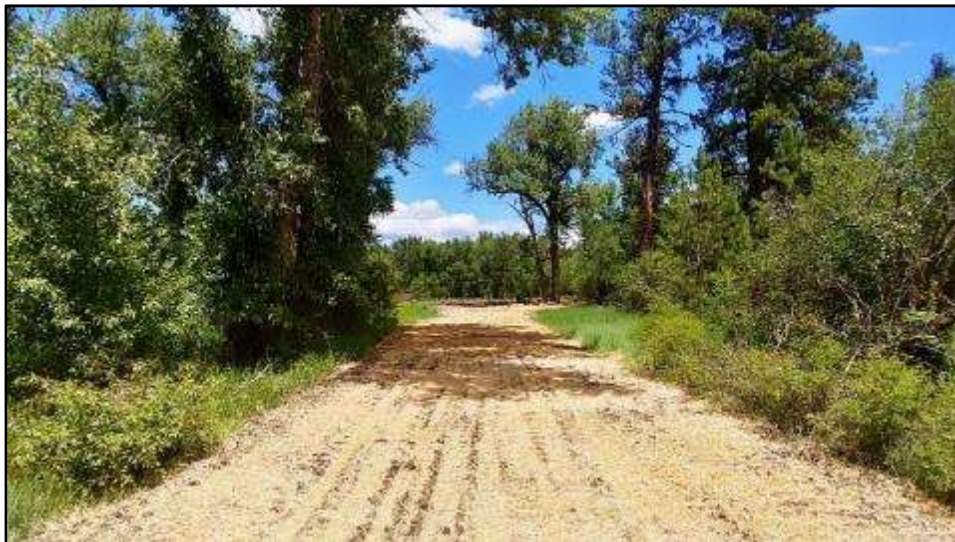
FIGURE 1 SEEDED AND MULCHED DECOMMISSIONED ROAD AT STATIONING MC 55+00
