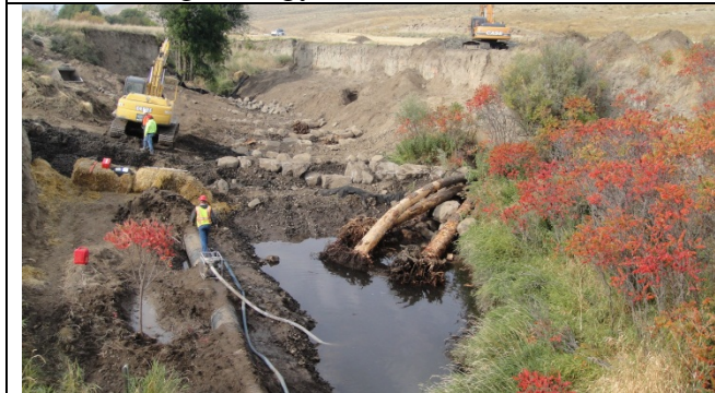
Generator pump used to reduce groundwater seep
