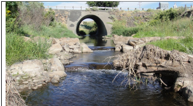
Notched cross vanes provide low flow channel
