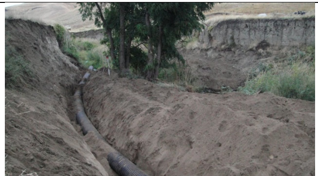
300' bypass pipe with all stream flow contained
