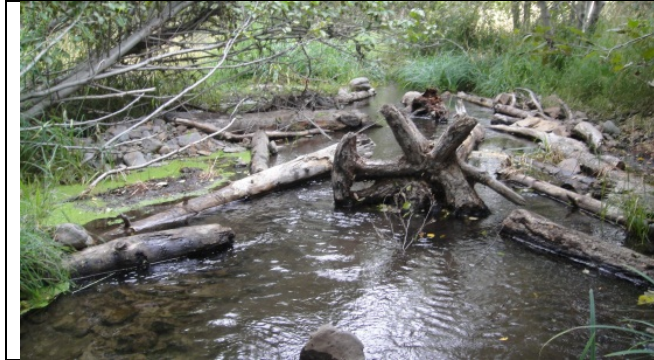
Conversion of glide to scour pool, reduced width
