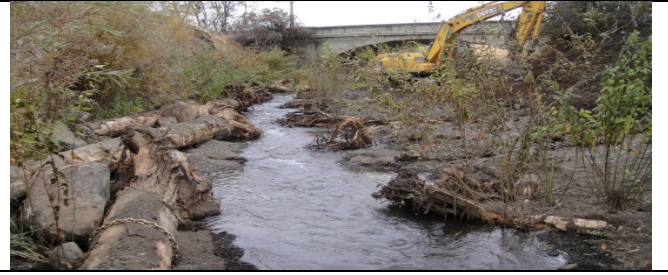
Protecting eroded bank, whips added
