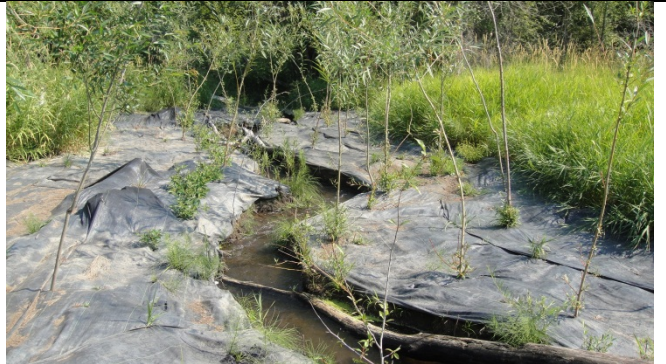
Sinuosity added and channel defined
