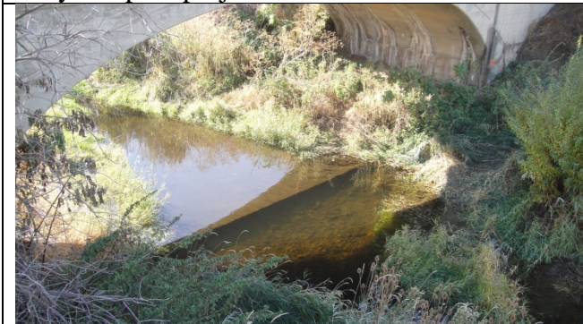
Rectification of 11' step, partial barrier
