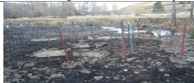
Fencing to restrict deer grazing on plantings
