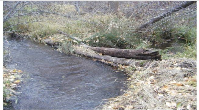
Upper plug created corner pool with undercut
