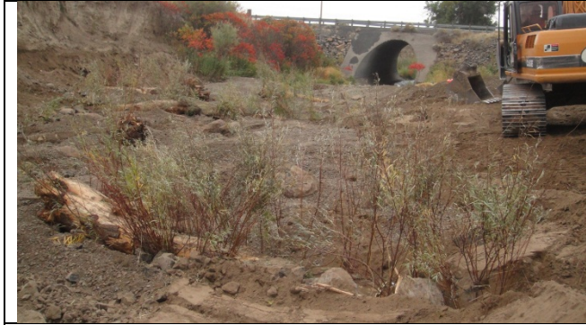
Roughened channel complete, ready to re-water
