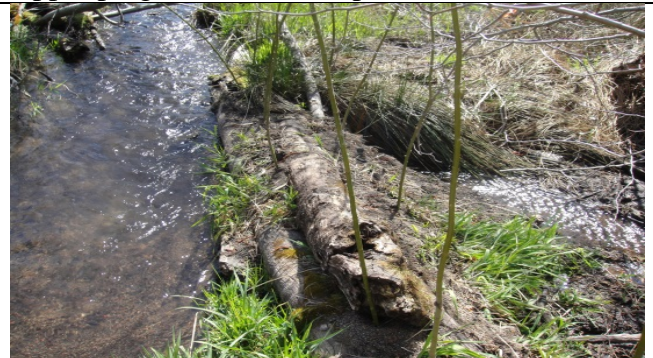
Plug planted for long term stability with whips
