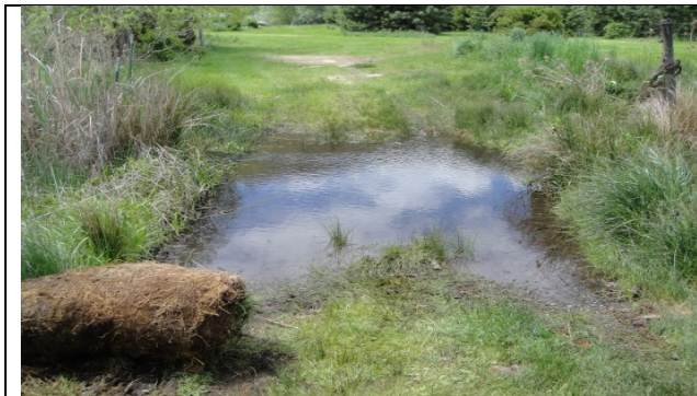
Sedge mat added to Wide glide crossing
