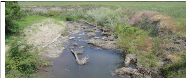
Debris deflecting flows into bank
