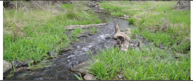
Forced thalweg to build velocity to form pools
