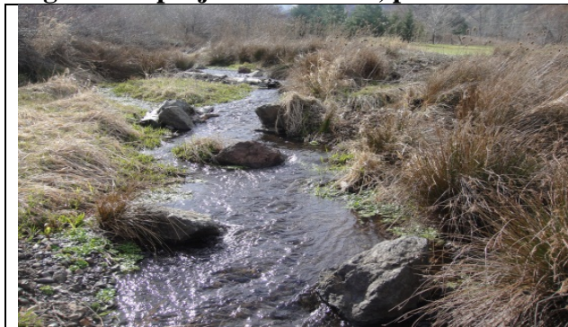
Riffle converted to sinuous riffle with pockets
