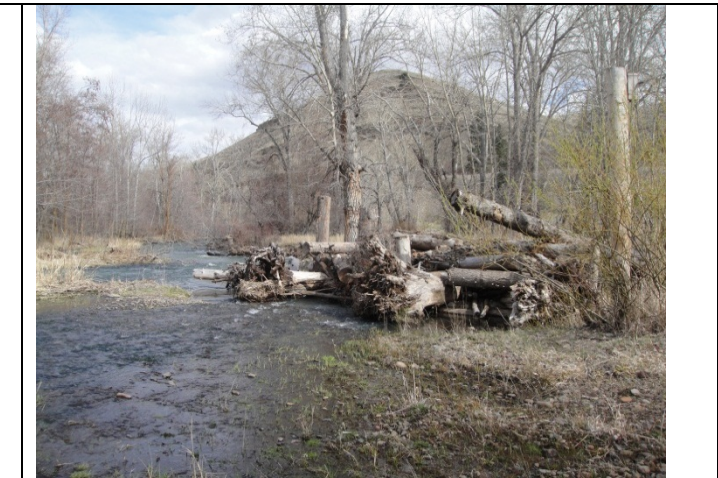
ELJ Constructed to protect bank from eroding
