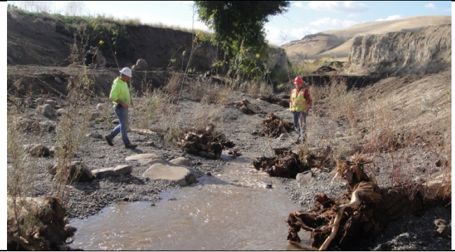
Slow re-establishment of flow to seal channel
