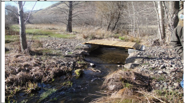
Drive thru crossing eliminated, bridge installed
