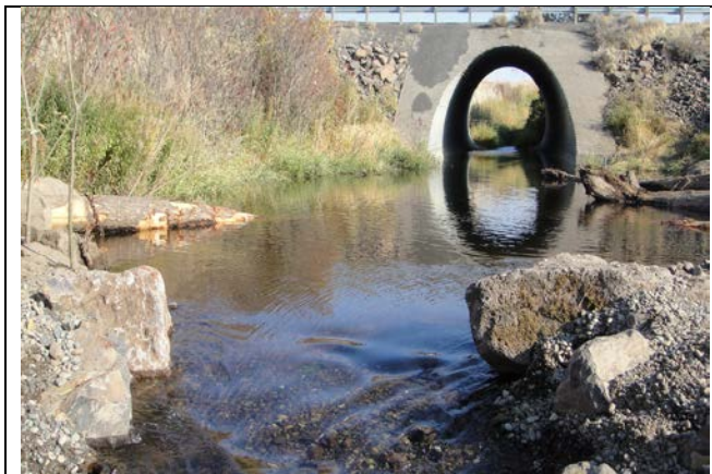
Elimination of 23" step at culvert achieved
