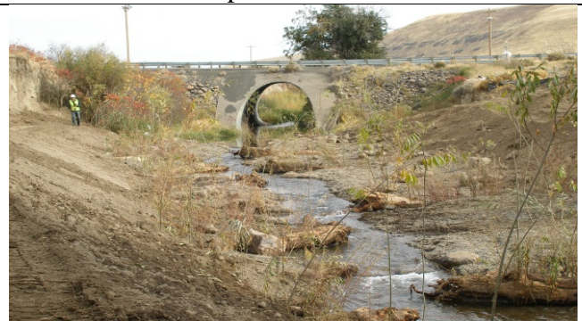
Sloped banks seeded with native grasses
