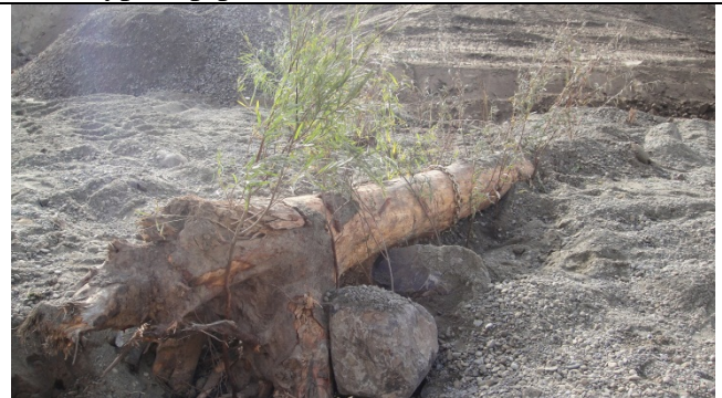
Stability methods for retaining LWD
