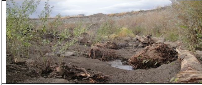
Willow whips put in LWD trenches, backfilled
