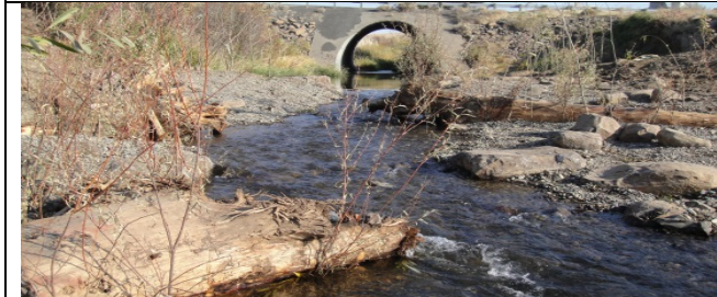
Placement of perpendicular LWD by cross vanes
