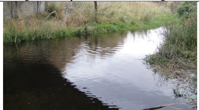
7" water depth in box culvert during low flows
