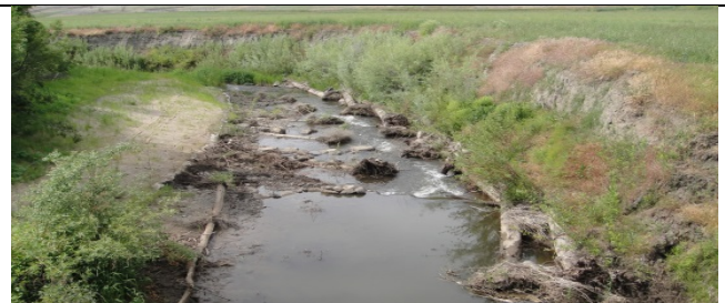
Debris removed from thalweg, placed on bank
