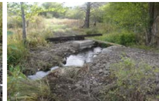
Hartssock Springs Bridge
