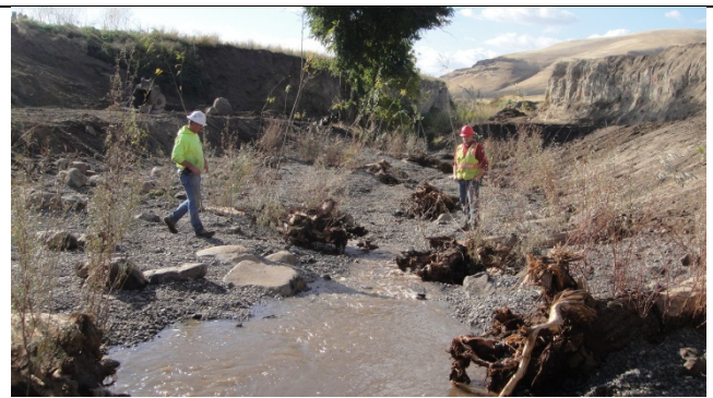
Slow re-establishment of flow to seal channel
