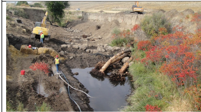
Generator pump used to reduce groundwater seep
