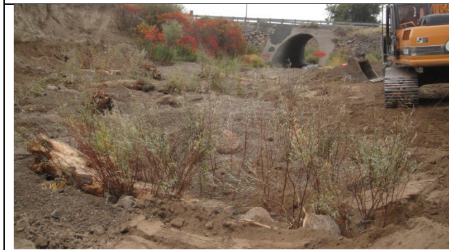
Roughened channel complete, ready to re-water
