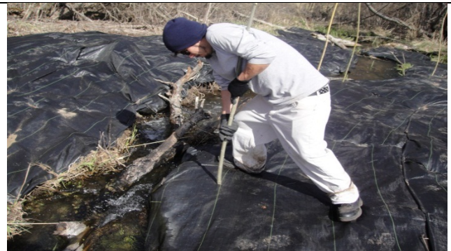
Full cuttings forced deep top reach ground water
