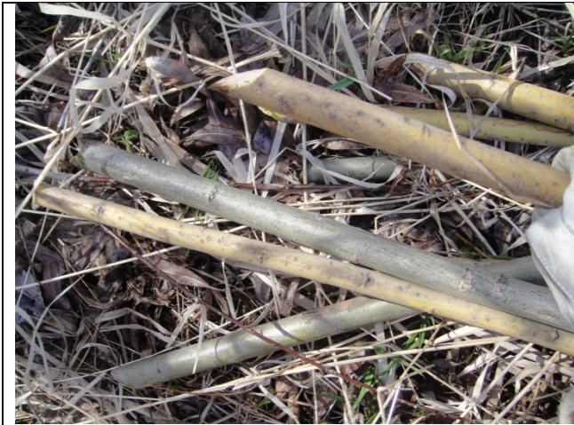
Cutting live Willow stakes near project site
