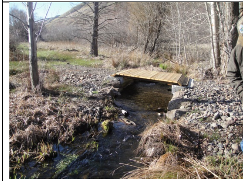
Drive thru crossing eliminated, bridge installed
