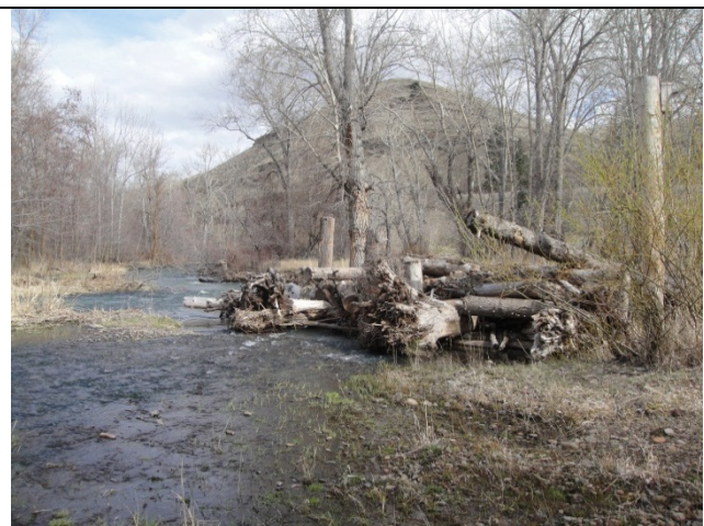
ELJ Constructed to protect bank from eroding
