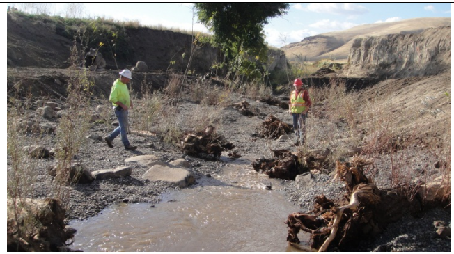
Slow re-establishment of flow to seal channel
