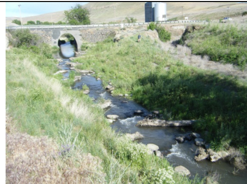
Blackberries Provided Substantial Undercut
