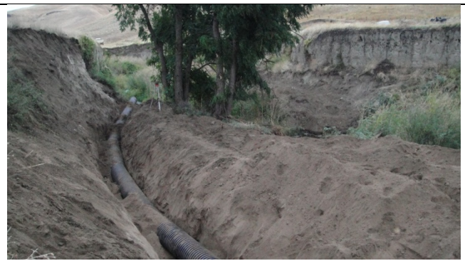
300' bypass pipe with all stream flow contained
