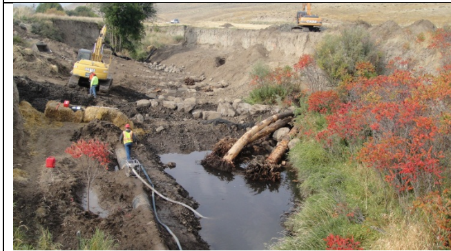
Generator pump used to reduce groundwater seep
