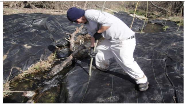
Full cuttings forced deep top reach ground water
