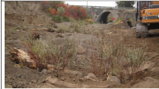
Roughened channel complete, ready to re-water
