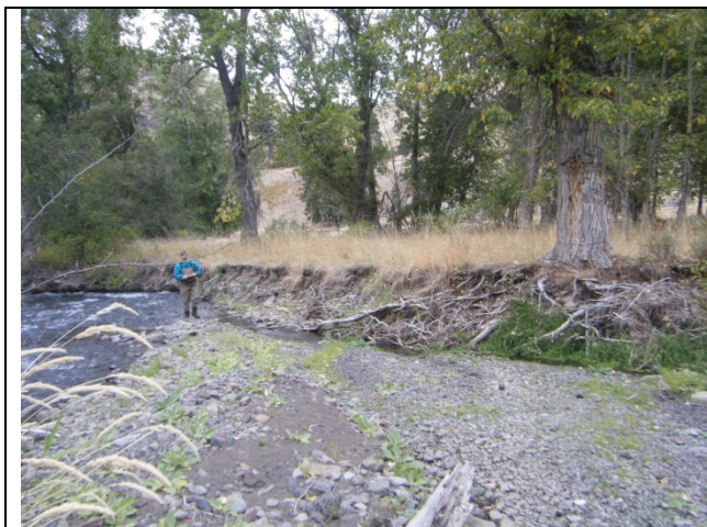
Actively Eroding Bank and High Terrace
