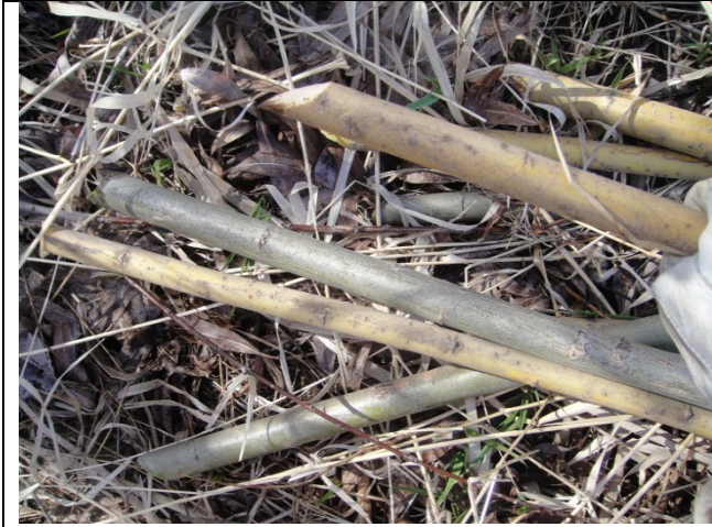
Cutting live Willow stakes near project site
