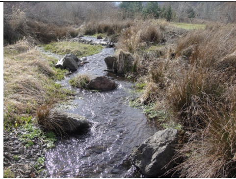
Riffle converted to sinuous riffle with pockets
