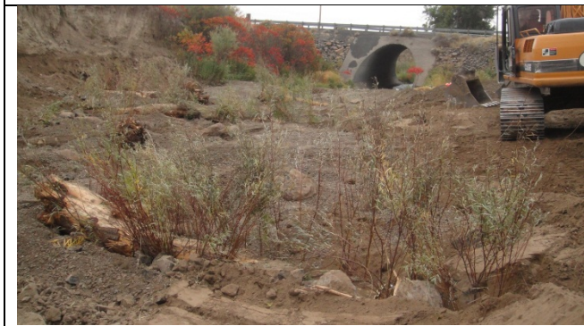
Roughened channel complete, ready to re-water
