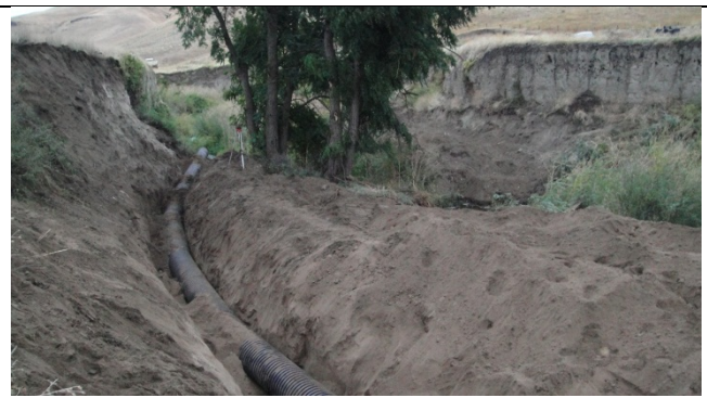
300' bypass pipe with all stream flow contained
