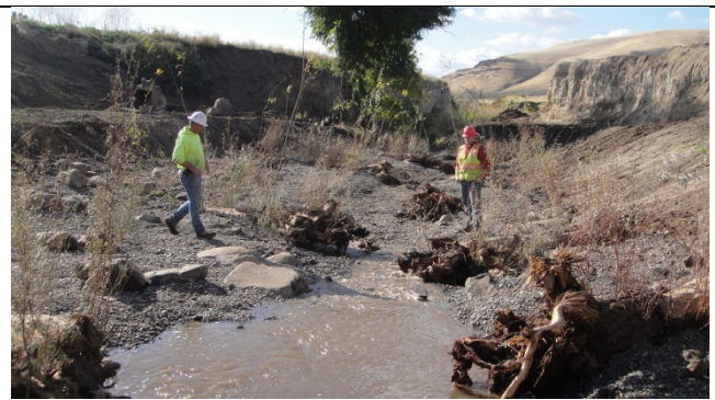
Slow re-establishment of flow to seal channel
