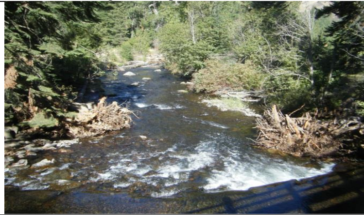
Overview from Panjab bridge after restoration
