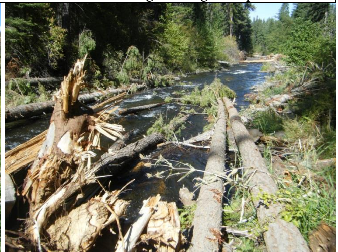
Converting a rapid to a series of pools
