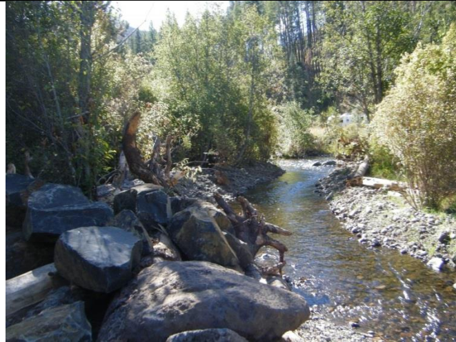
Additional bank protection near braid inlet
