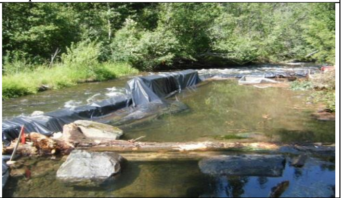
Much emphasis on turbidity control via. isolation
