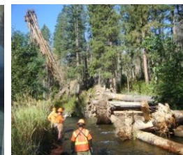
2013 Completed Project 2014 Planned Project, Tucannon River
