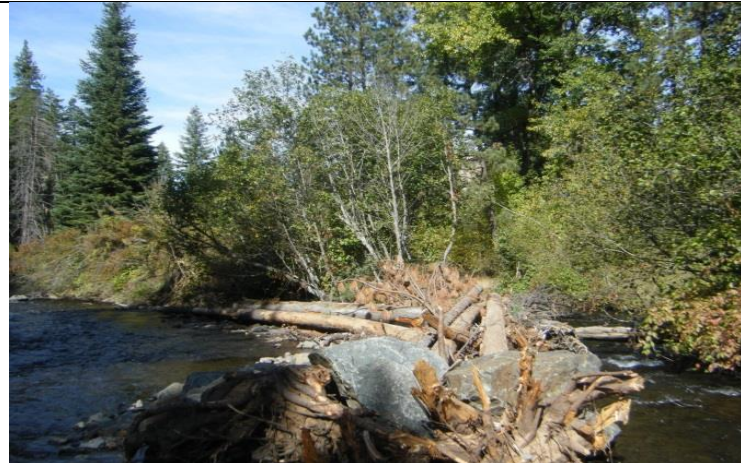
Extended apex to promote split channel wishbone
