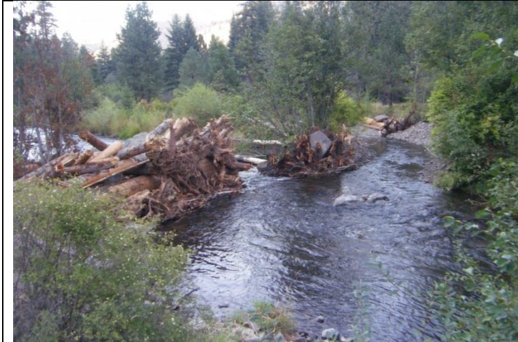
ELJ deflector and apex jam to create braided channel
