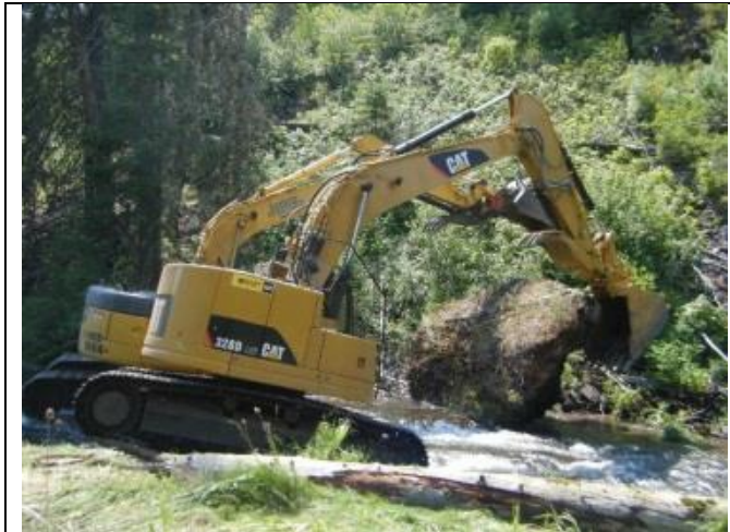
Relocating 14' boulder from bank to mid-channel
