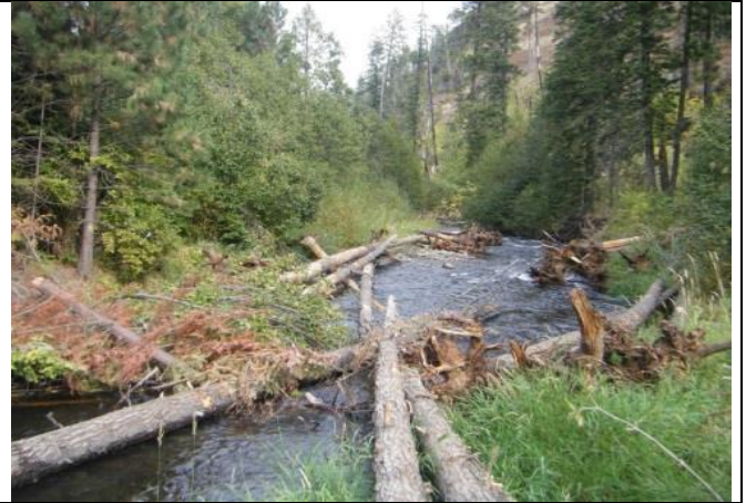
Undercut created using existing & imported wood
