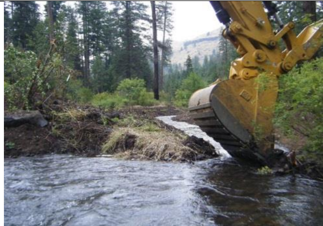
Slow activation of secondary channel, reduces silt
