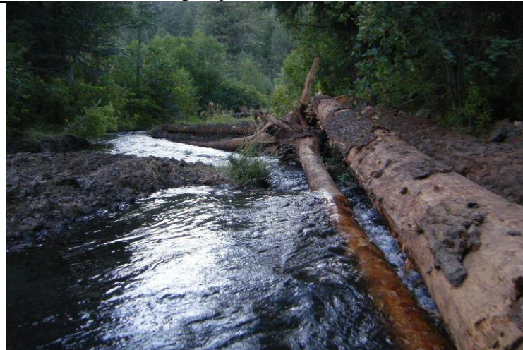
Overhead cover provided by undercut bank simulation
