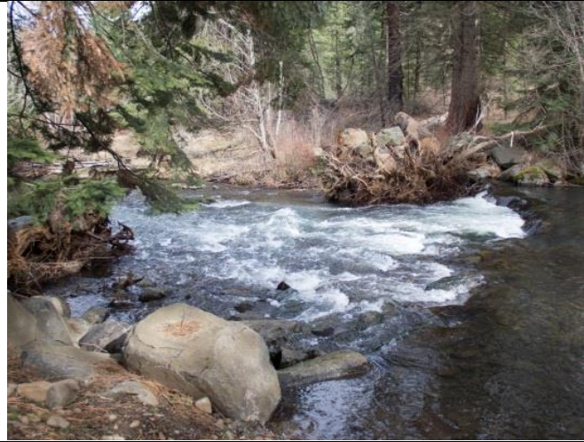
Roughened channel and notched cross vane
