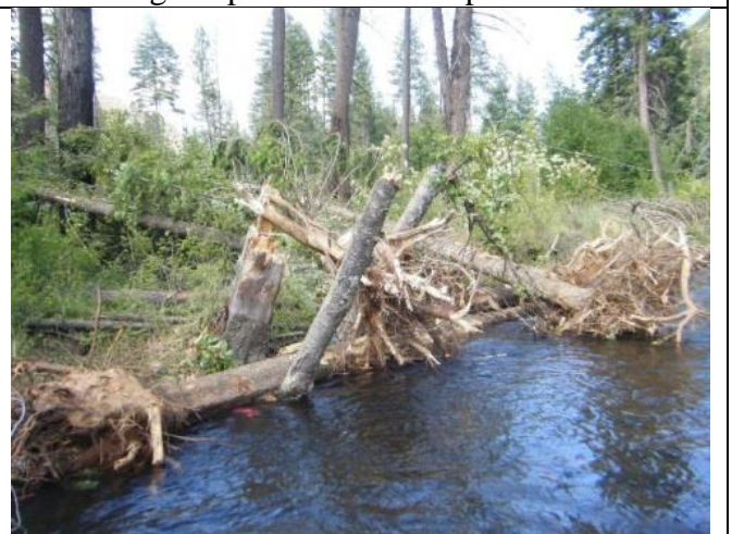
Using existing dead trees as pillars to hold LWD
