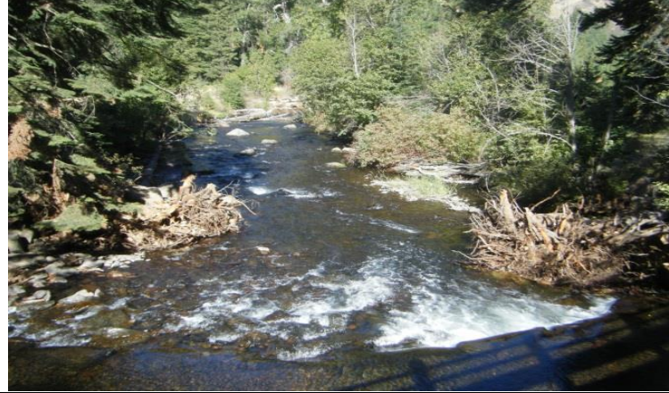
Overview from Panjab bridge after restoration
