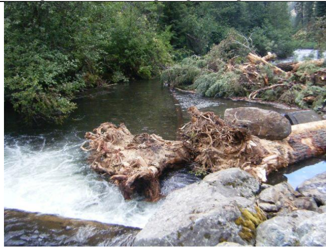
Root wads and tail out ELJ to rectify passage
