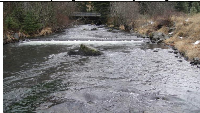
Channel spanning log passage concern, Panjab
