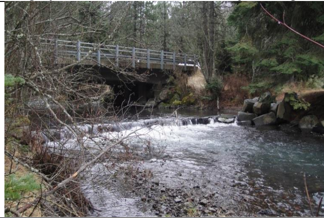
Cross vane, passage concern, Panjab Bridge
