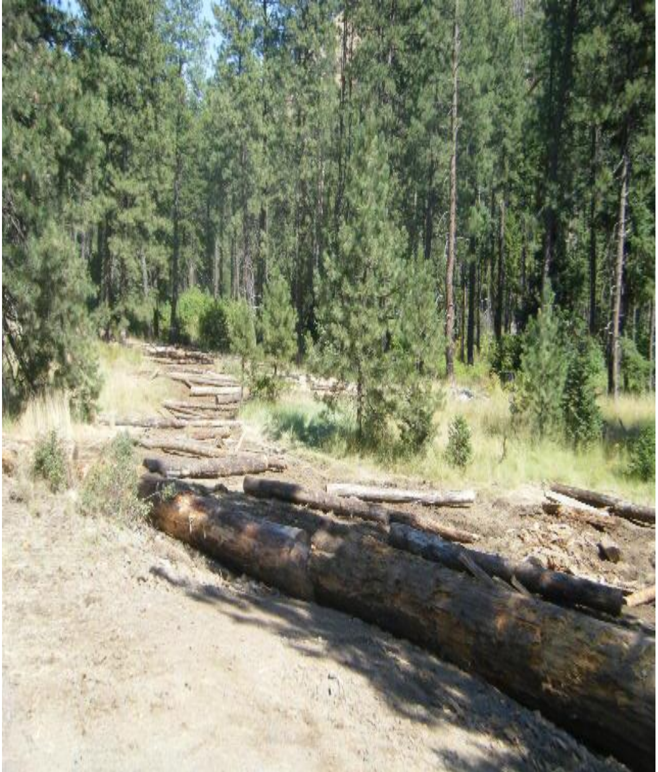
Figure 28. Decommissioned roadway detail, following implementation, recovery promotion
