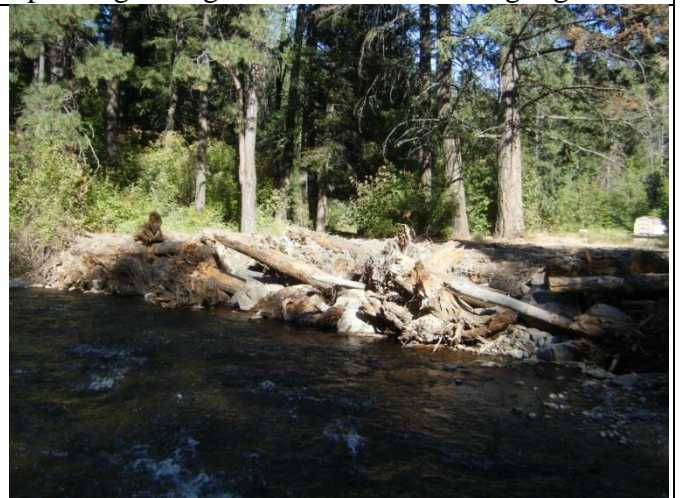
Stream bank ELJ to protect Wooten infrastructure
