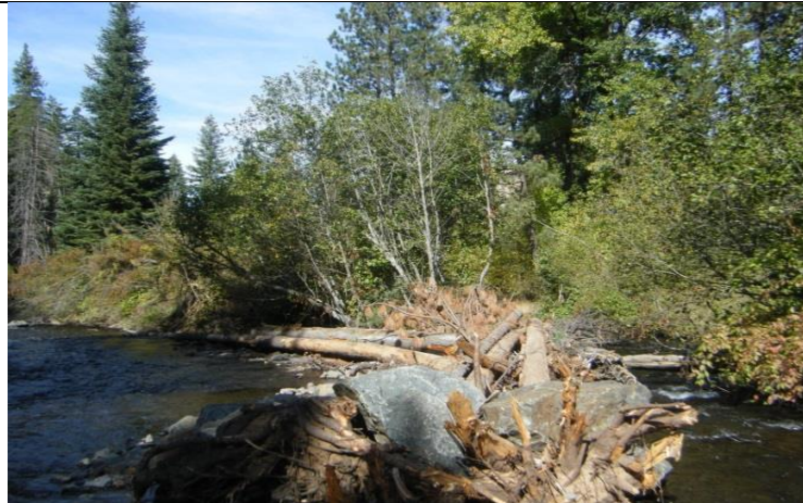
Extended apex to promote split channel wishbone
