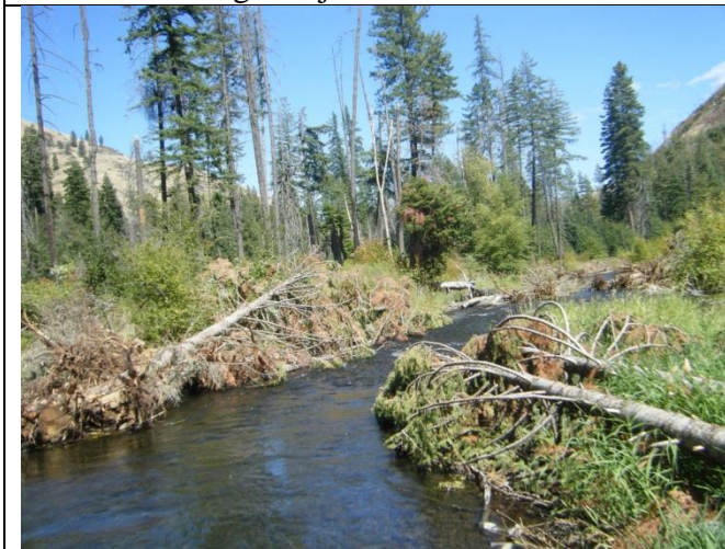
Green tops placed in channel for juvenile cover
