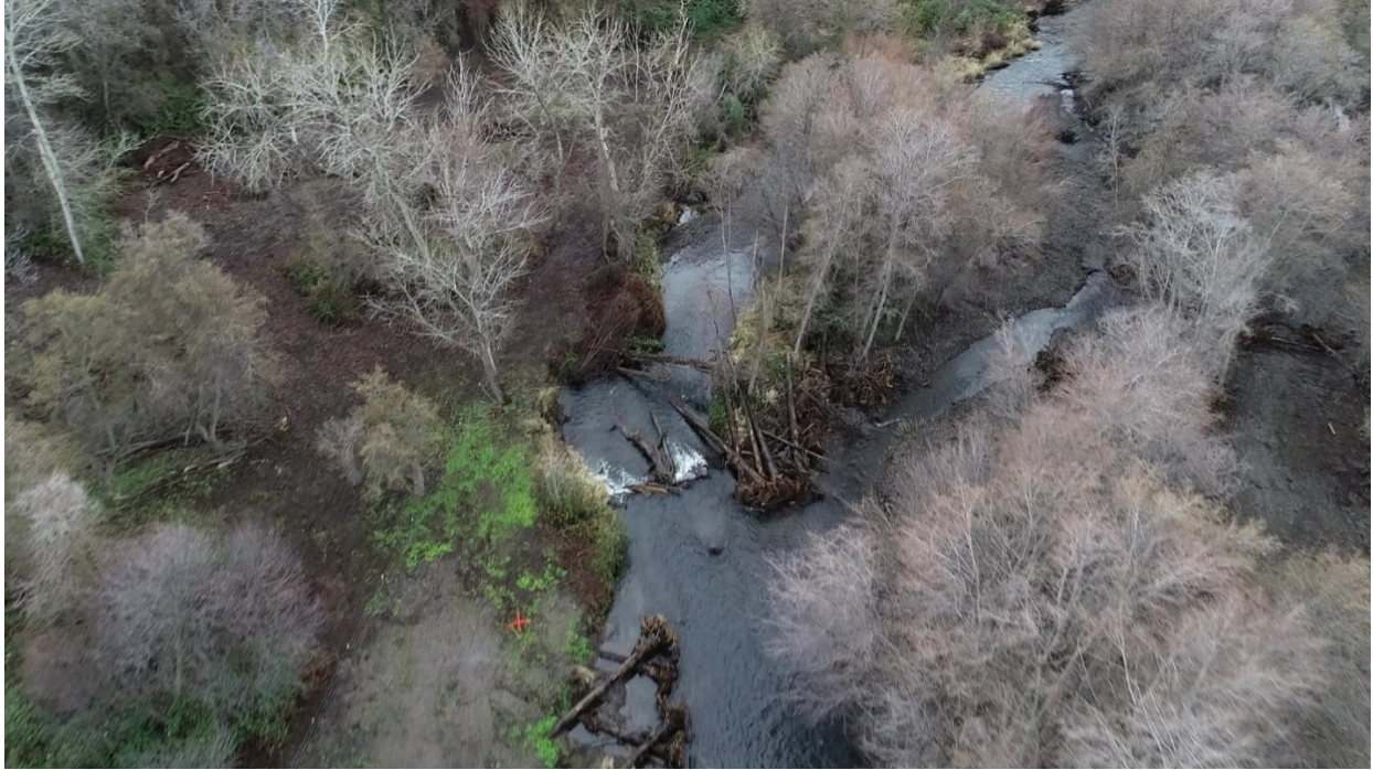
Large wood structures installed in PA27/28.1 during Phase 0.5 implementation. Image was taken from a drone survey on February 2021.
