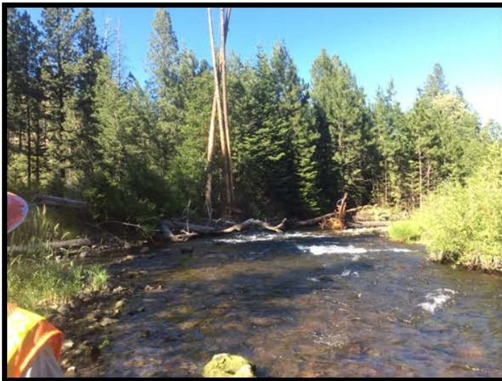
Figure 15: Project Area 3, Tucannon River channel complexity placed using Vertol helicopter, July 2014 by the Confederated Tribes of the Umatilla Indian Reservation Tucannon Program. (Upper) Pre-project condition of the meander jam and channel spanning structure built below Little Tucannon confluence, ground photo left and aerial image right. (Lower left) Logs being placed by the helicopter, (lower right) final product captured in September 2014. Note the natural jam in the lower right of the lower right photo, it has been used as a reference for channel spanning structures in the Tucannon.
