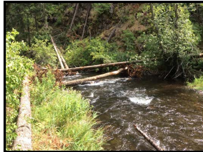
Figure 17: Project Area 3, Tucannon River channel complexity placed using Vertol helicopter and conventional methods, July 2014 by the Confederated Tribes of the Umatilla Indian Reservation Tucannon Program. Upper left, log channel spanner placed using conventional excavator for the purpose of providing structural stability near the bottom of the project reach. Note the large rock placed on top of the wood elements to provide ballast to the structure during high flow. Lower left is a pre-structure view of the right upper and lower images in post project.
