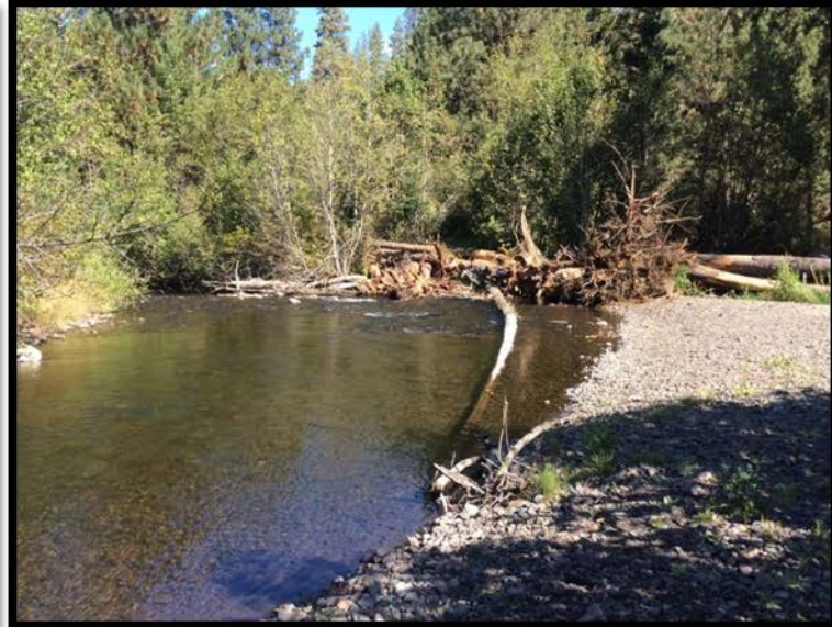
Figure 11: Project Area 1, Tucannon River channel complexity placed using Vertol helicopter July 2014 by the Confederated Tribes of the Umatilla Indian Reservation Tucannon Program. Upper left, preplacement of channel spanning structure, (Upper right) post project placement of channel spanner. Lower left, the placement of channel meander jam in progress, (lower right) completed channel meander jam. All photos are representative of structures placed by helicopter.
