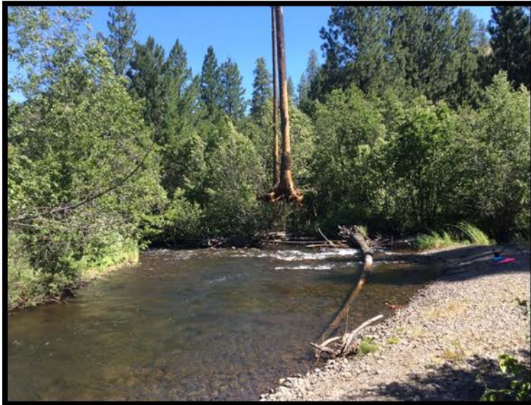
Figure 11: Project Area 1, Tucannon River channel complexity placed using Vertol helicopter July 2014 by the Confederated Tribes of the Umatilla Indian Reservation Tucannon Program. Upper left, preplacement of channel spanning structure, (Upper right) post project placement of channel spanner. Lower left, the placement of channel meander jam in progress, (lower right) completed channel meander jam. All photos are representative of structures placed by helicopter.
