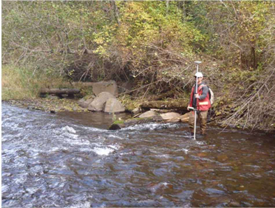
Figure 2-4. Photograph of existing LWD and boulder groin structure.
