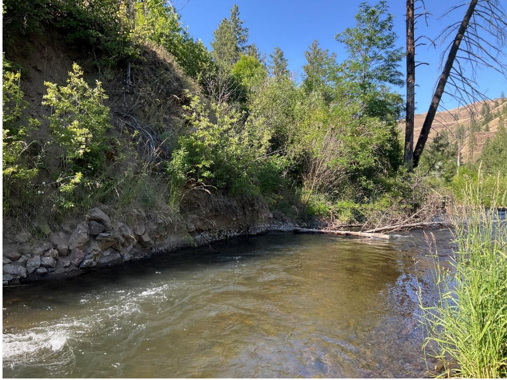
Photo Point 31: Downstream view of Tucannon River, along high eroded and incised banks (river left); view N.
