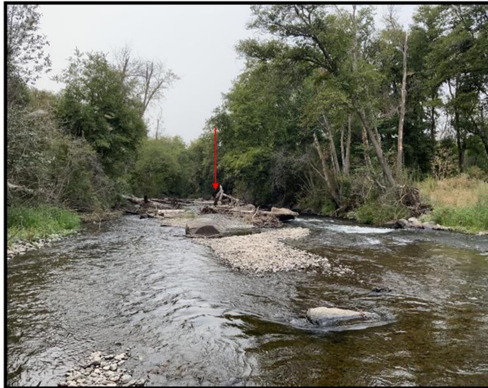
Figure 26-11: Project Area 26 Phase II pre (upper left) post project 2021 (upper right), post 1 flow summer 2022 (lower left) and post two flow events winter 2023 (lower right) above a apex spanning structure designed to aggrade the channel bed and increase channel meander and floodplain inundation over time. During the 2021-22 winter/spring flows which were moderate the structure was largely buried in gravel (lower right) and channel migration to river left began undercutting the left bank.
