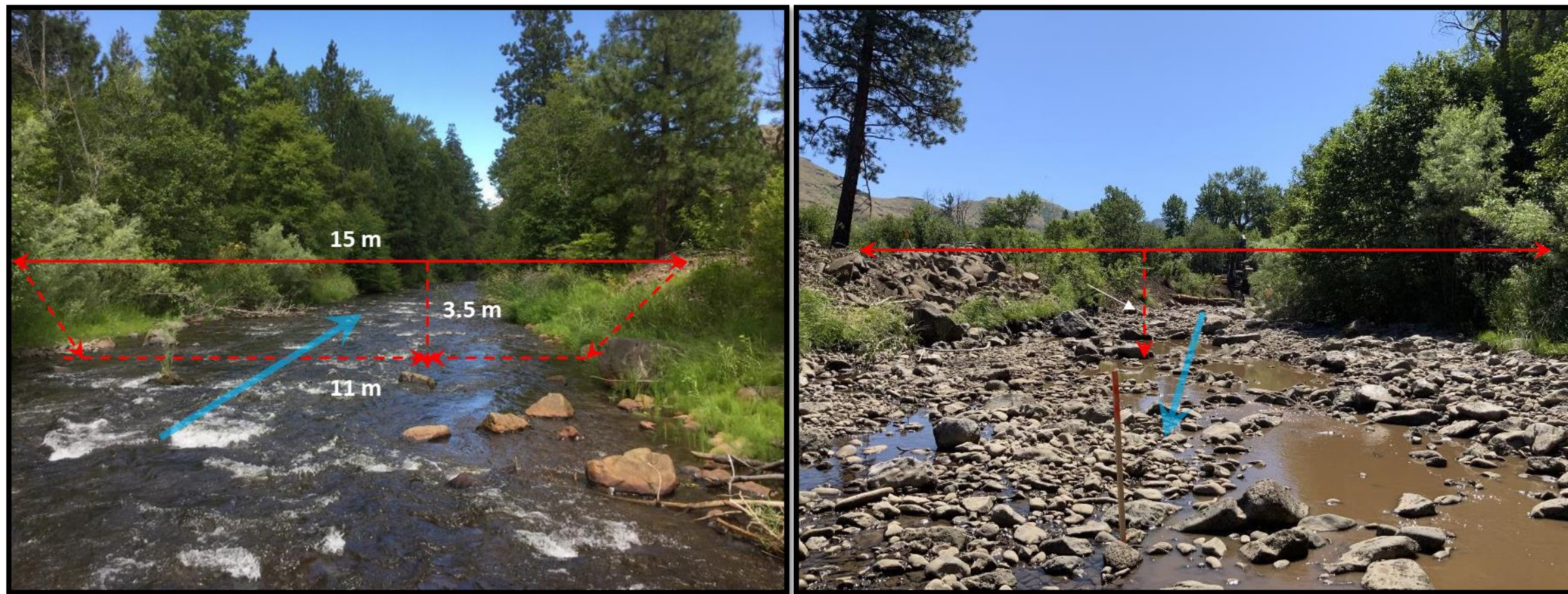
Figure 13-2: PA13 levee removal and channel plug location 2021 to post Phase I implementation in 2022. Upper left illustrates the river confined on the right by a steep rip-rap protected bank on the right and the valley wall on the left illustrating a confined bank full geometry which leads to unnatural stream power for the Tucannon and the stream bed exposed during construction dewatering (upper right). Removal of the right bank levee and rip-rap reduces the depth of bank full geometry (lower right) bring stream power back to values predicted based on valley metrics. The blue arrows indicate flow direction as well as flow paths during high water events.
