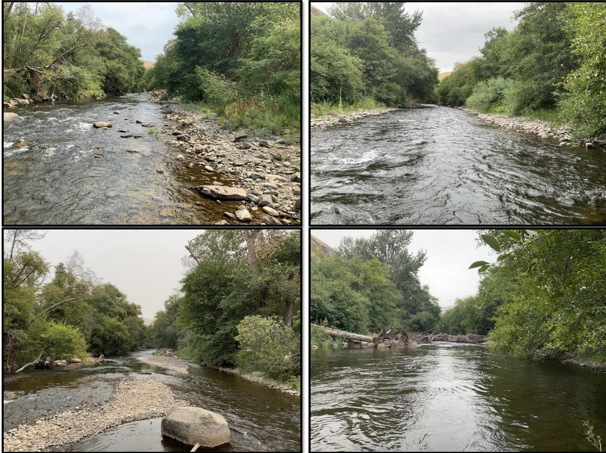
Figure 26-12: Project Area 26 Phase II pre (upper right & left) and post (lower right & left) plain bed reaches treated LWD structures to improve gravel deposition bar formation and habitat unit complexity. The two upper reaches were treated in 2021 and the lower two images are the result of a single year of moderate seasonal flow (~1Yr return interval).
