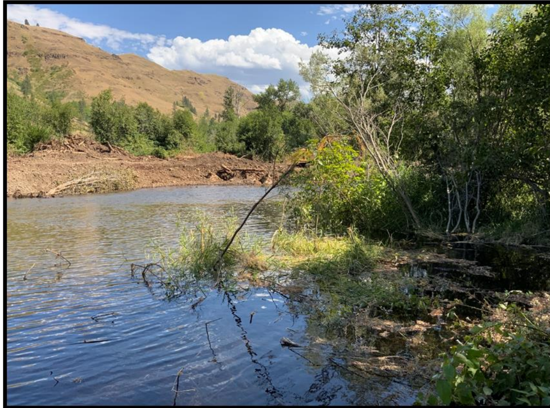
PA13-12: PA 13 Phase I side channel (upper right & left) and off channel units (lower left and right) created through removing confining features and channel plugs.
