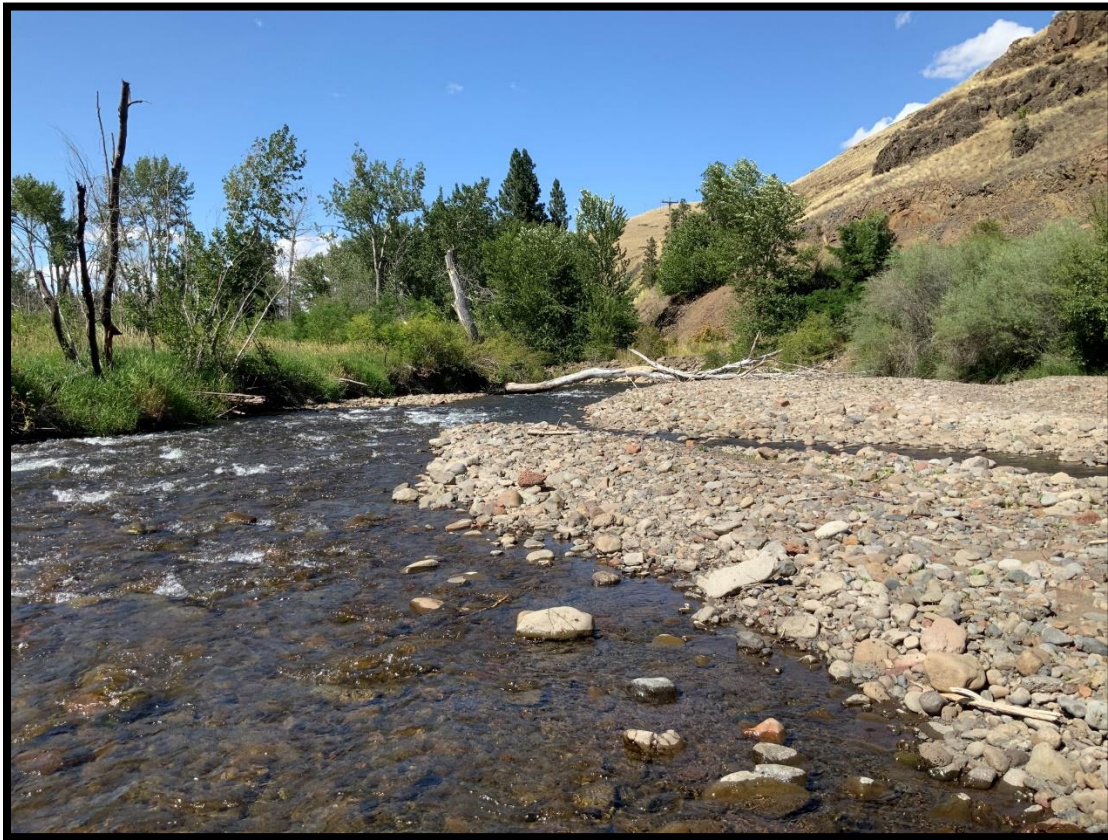
Example channel conditions being targeted for additional channel roughness under the PA15 Phase II design.
