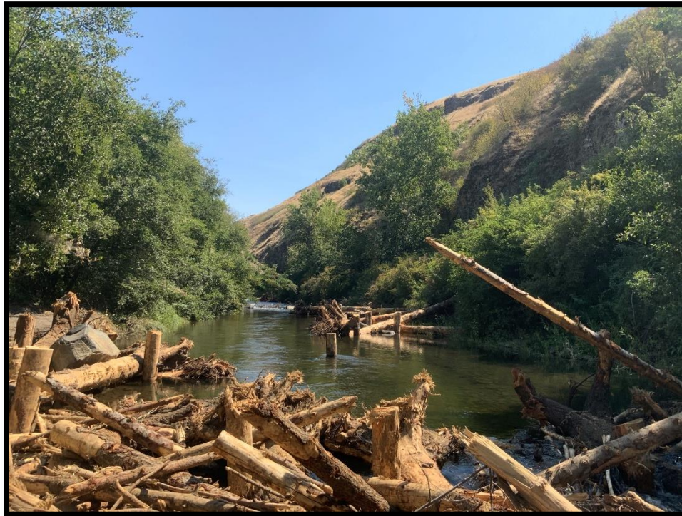
Figure 25: Pre (upper) / post (lower) project images in a plain bed -reach treated with LWD structure to increase channel complexity and floodplain connectivity at PA26 in 2021.
