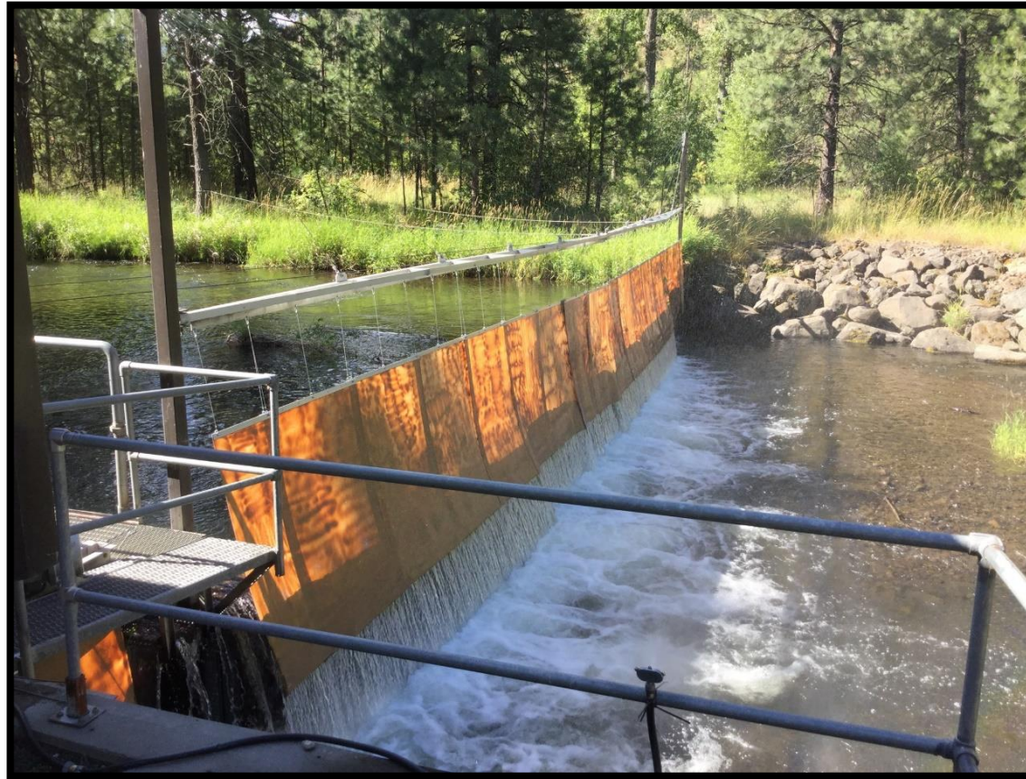
Figure 6: Tucannon River Project Area 13 pre-project conditions in 2018. The upper left image is the Tucannon Fish Hatchery weir and fish trap located at the upper most end of the project area. The project reach is described as a combination of plain bed riffle and rapids (lower left and right images) caused and maintained by river levees and riprap. The upper right image shows one of the river levees being removed in 2022 as part of the restoration project design for this reach.
