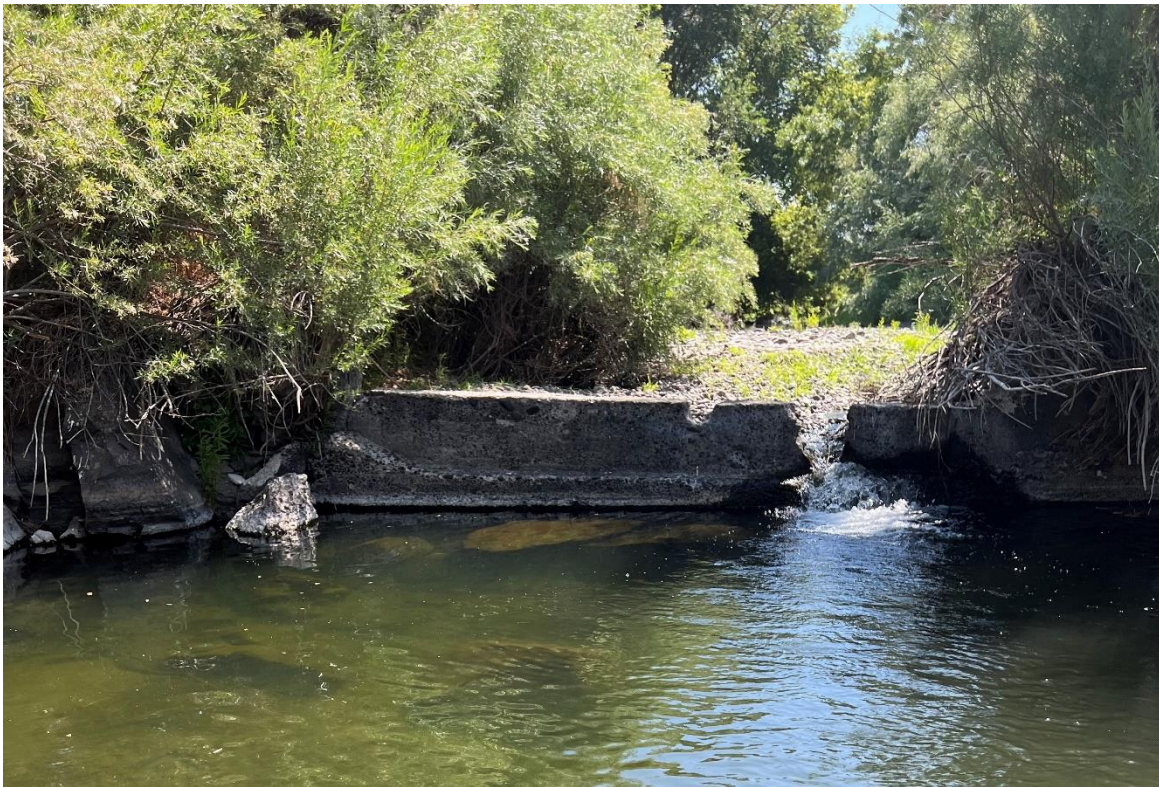
Figure 1-3. Existing Conditions at Peterson Dam Structure
